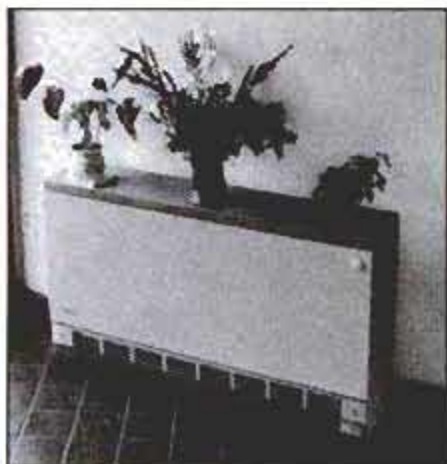
Stiebel Eltron storage heater installed in a home. Units are expensive, but savings from off-peak power rates add up.
