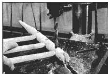
Clear holes to bottom using a 1/2-in. bit.
