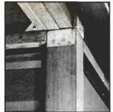
The detail (left) shows two upper rails joining a capped post. Detail (above) shows a metal post-and-beam tie. Note corner of the joist hanger (top left).
