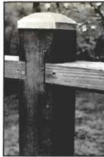
The detail (left) shows two upper rails joining a capped post. Detail (above) shows a metal post-and-beam tie. Note corner of the joist hanger (top left).
