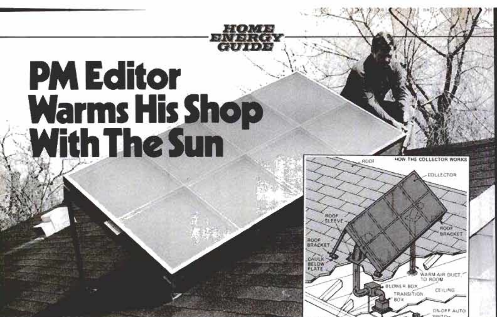
Independent roof system includes the 4x8-ft. collector, blower and thermostat.
