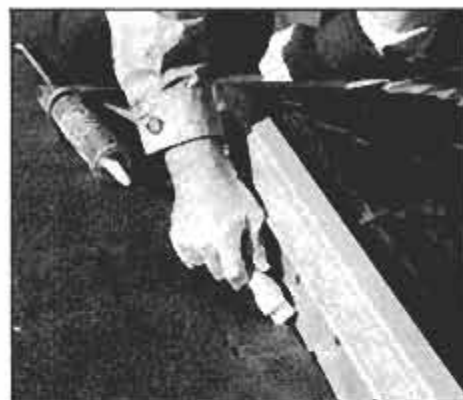
Stiff brush cleans dirt from cracks, so caulking can adhere to both materials.
