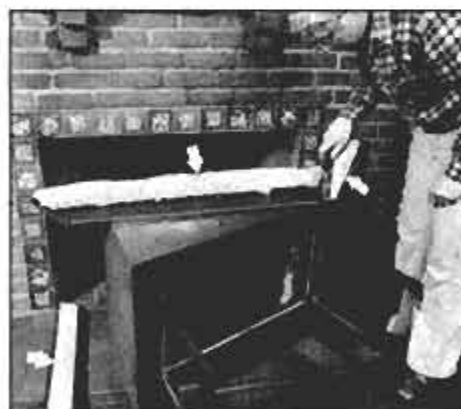
Fireplace-surround trim (arrows) is installed using screws supplied. Three pieces come with insulation affixed.
