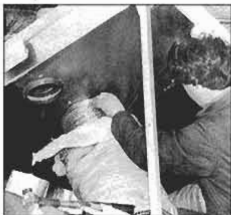
Flexible duct is pulled up around collar (flange) and is held by clamp. Next, insulation is positioned and secured with duct tape. Under normal conditions, flexible ducting outdoors should last five years.
