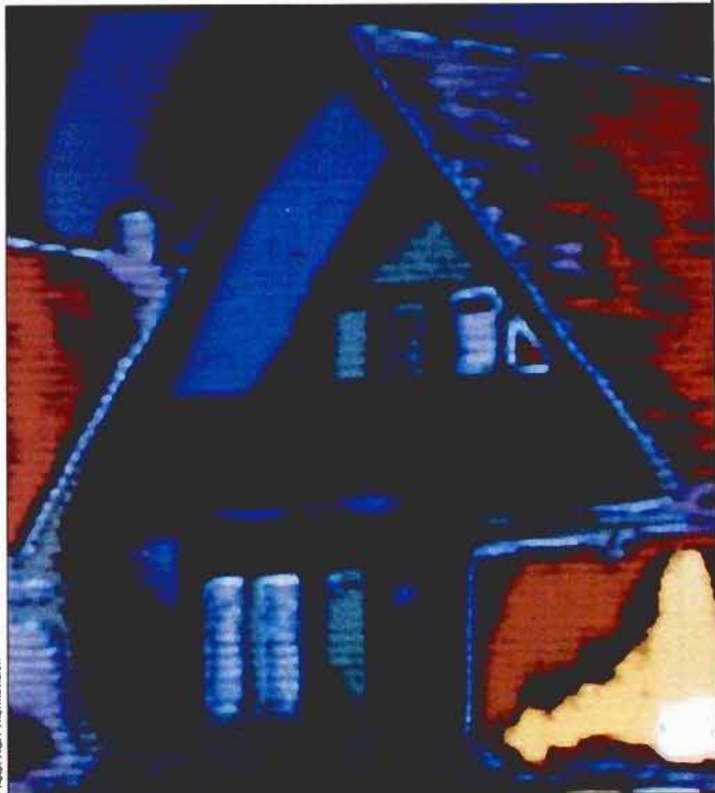
Thermogram is a photo taken with infrared film that registers heat rather than light. Red areas show where heat is escaping
