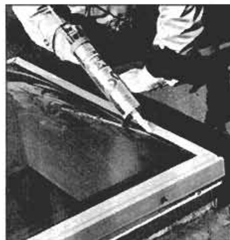
Clear caulk seals joint between acrylic bubble and the aluminum skylight frame.
