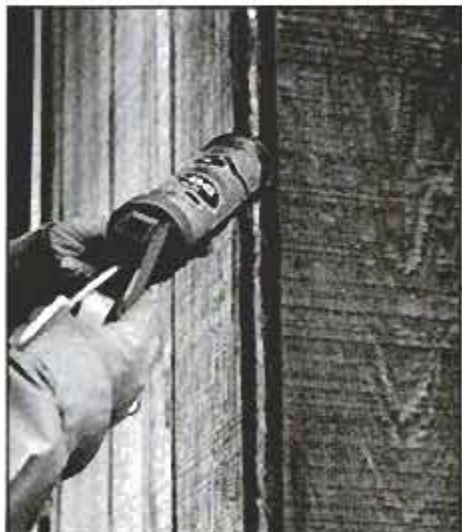
Outside corner where side walls meet can be caulked with clear acrylic copolymer.
