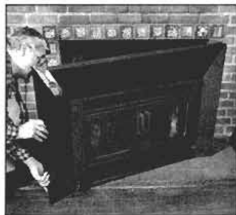
Screws holding first two trim pieces are only finger-tightened until third piece has been aligned and attached to unit.
