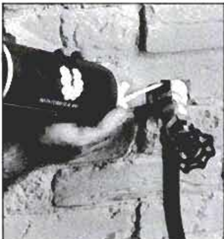
Foamed urethane insulation from aerosol tube can seal larger gaps, like this rough opening around hose bib in the brick foundation. Apply several thin coats.
