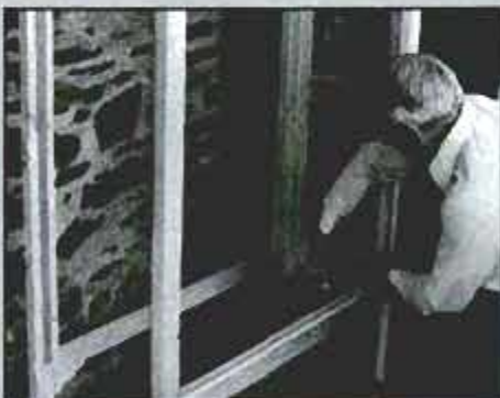
Start construction by attaching cabinet frame to side panels with \frac{3}{4} -in., No. 10 flat-head screws. Screws are countersunk in cabinet frame's vertical cleats.
