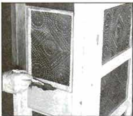
Brush on a stain/sealer after sanding edges lightly and taping around tin panels. Alternately, you may apply polyurethane varnish alone to preserve natural color.
