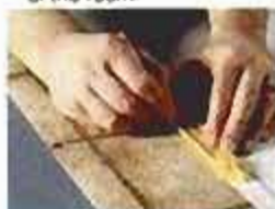
2. Transfer the pattern to your new floor.
