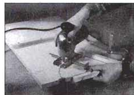
2 Make cut with sabre saw and pivot guide. Apply tape to cut line and support waste with clamp to prevent splintering.
