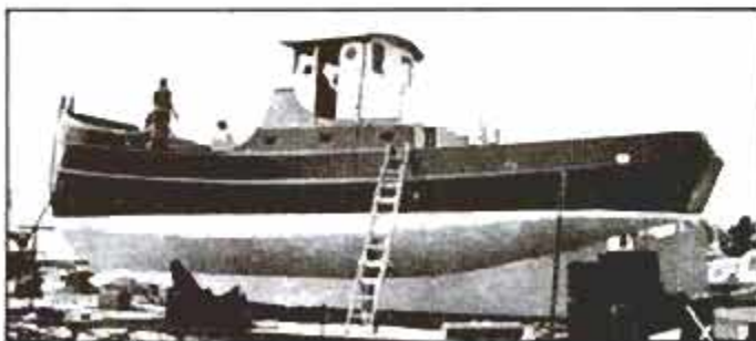
Shown under construction, unusual hybrid hull has stubby keel.
