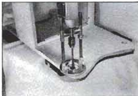
6 After both panels are joined to sides, bore hinge-peg holes. Use Portalign tool or other drill guide to ensure accuracy.
