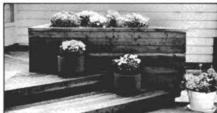
The built-in planters at the steps serve as railings while displaying blooms or greenery. Rather than being cantilevered over the step, both are supported from below (see the drawing).
