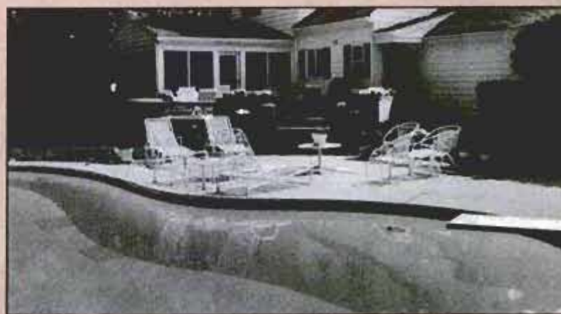
View from across the pool shows how deck is designed to follow the contours of the house, and visually link it to the pool.
