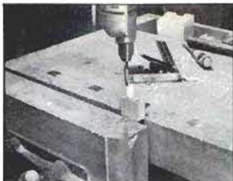
8 Bore dowel holes to desired depth; note masking-tape depth stop on the bit.
