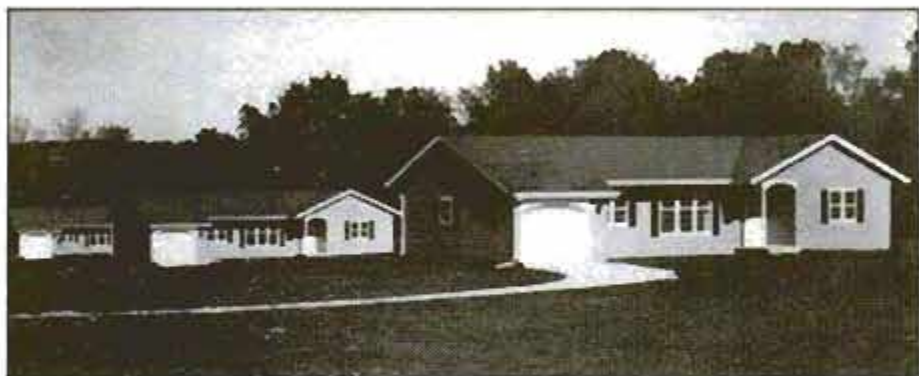
Test homes were built near Madison, Wis., to furnish data for Owens-Corning's EPDS program. Full-scale tests showed advantages of double-stud wall construction.
