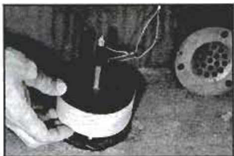
When heavy rains threaten, remove drain cover and place alarm device in position.
