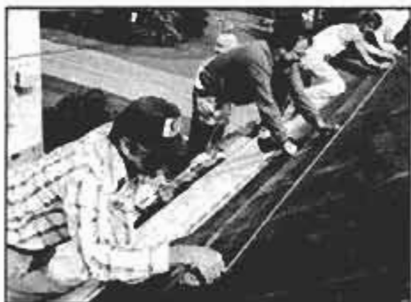
An in-process photo of shingling job shows three courses in place and a fourth course in progress. Note that drips (tab cutouts) are staggered in adjoining courses.
