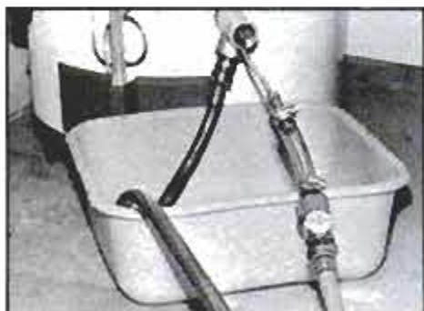
Attach drainage garden hose (left) to lower basin-tee outlet with second close nipple and coupling. Most flush water can be drained directly into a basement drain.
