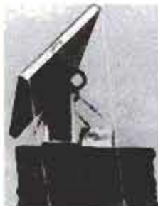
A chimney-mounted solar panel can be adjusted for best sun angle from ground.
