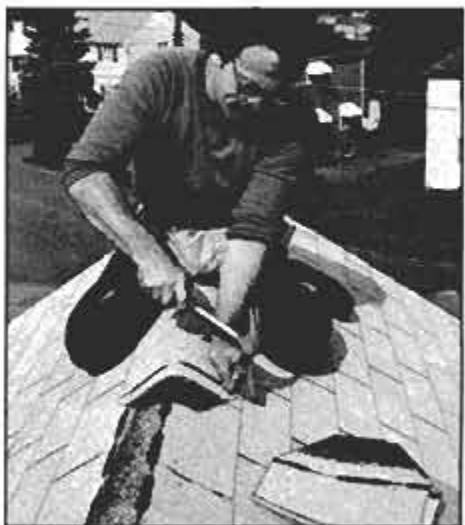
The Boston ridge is the most commonly used type of ridge cover. It's made of one-third pieces of shingle, lapped 5 to 6 in. for double coverage, and blind-nailed.
