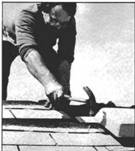
You may have to trim shingles abutting vents and such. Nail as possible. Set shingle; cover the nailheads with cement.
