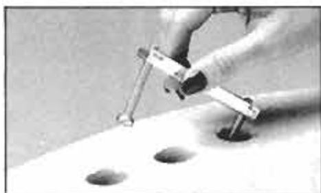
Insert one side of U-shaped tiebar assembly in outside basin hole. Maneuver until same screw comes up other outside hole.
