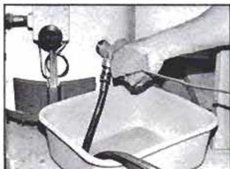
Block the probe hole with a sponge or cloth to cut flush water gushing through hole. Use a pan as shown, because some water will escape as probe is maneuvered.
