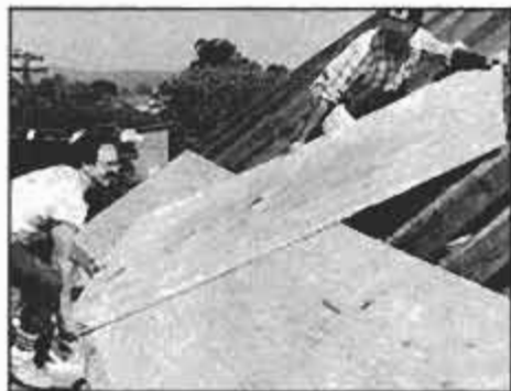
Plywood sheathing should be installed with its face grain perpendicular to the rafters. End joints are centered over the rafters.
