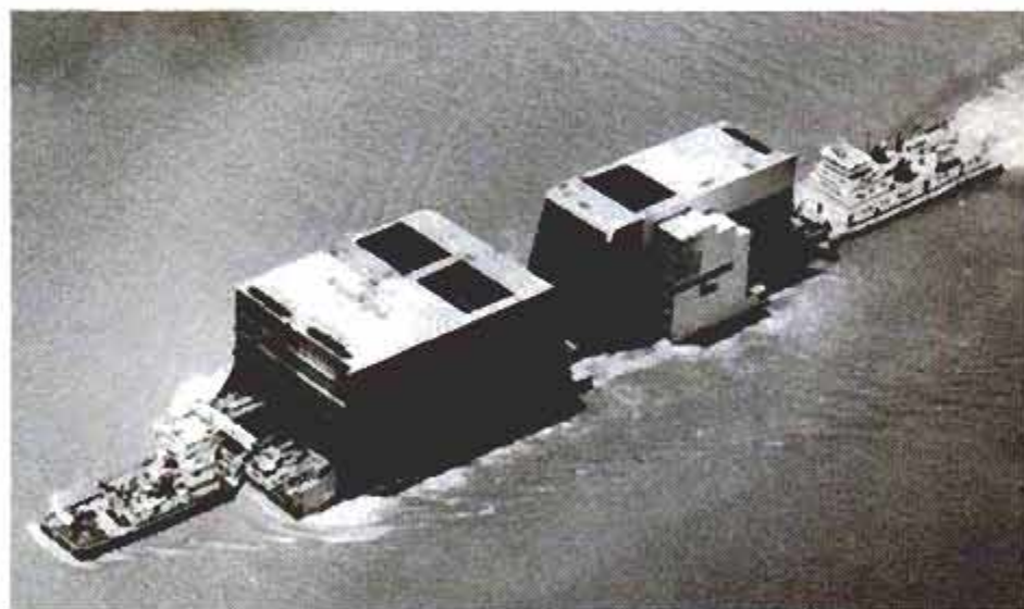
Completely fabricated in a French shipyard, generating plant for Vanceburg, Ky., was carried transatlantic by a special ship and broken down for the upriver tow.
