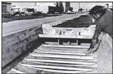
Pressure-treated 2x4s are notched to fit, secured with stainless self-tap screws.
