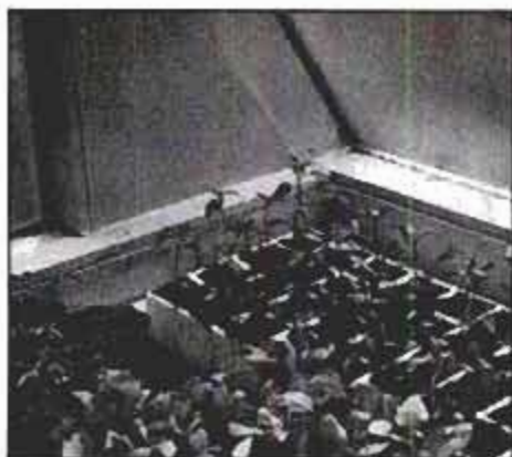
Corner detail of the greenhouse shows the sill plate, 2x6 stud and sheathing. The plant flats rest on removable ledges.
