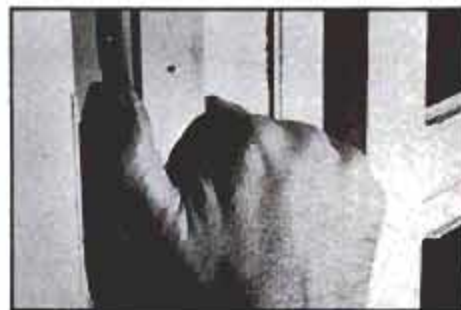
11 Weatherstripping should expand as door is opened if it's installed while sufficiently compressed to make a tight seal.
