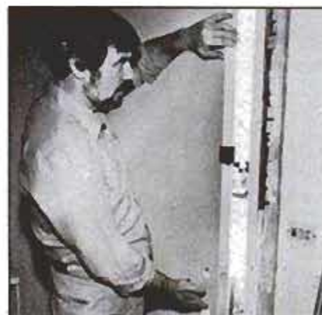
8 Retainer brackets hold unit firm for installation. Remove bracket screws. If the frame is square, door opens easily.
