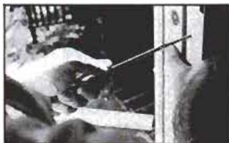
9 Install 11 screws in the sides and top of the door frame. If the screws are overtightened, the frame could be distorted.
