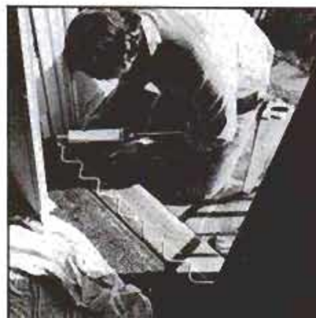
6 After all fitting adjustments are made, lay a zigzag bead of caulk across the sill. Then, permanently install the frame.
