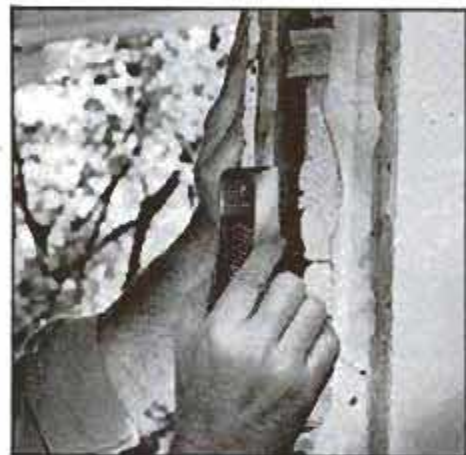
3 Use a Surform tool or plane to remove irregularities in old door jamb that might hold new door frame away from the wall.
