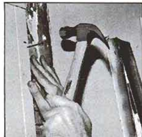
7 Nail the door frame to the jamb, using 1½-in. nails provided in the kit. Predrilled holes make this an easy step.
