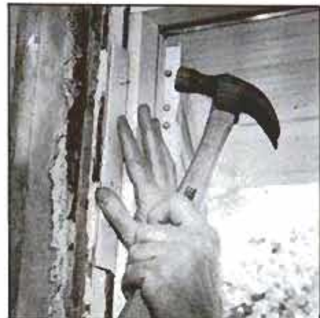
5 Use shims between jamb and frame to ensure a snug fit and to bring the jamb plumb. Nail shims over the mortises.
