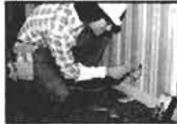
Installation of wiring—residential and industrial.
