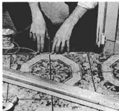
Conceal circuit line under the door's saddle. Keeping circuit line close to the floor will minimize needed wire.
