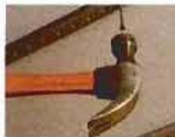
1. Nail up tracks.
