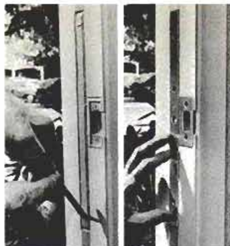
You can reinforce the door jamb by letting-in a metal plate. This heavy-gauge metal security plate costs $10.28 and is available from Keefe Lock Co., 1324 Parkside Ave., Trenton, N.J. 08638.
