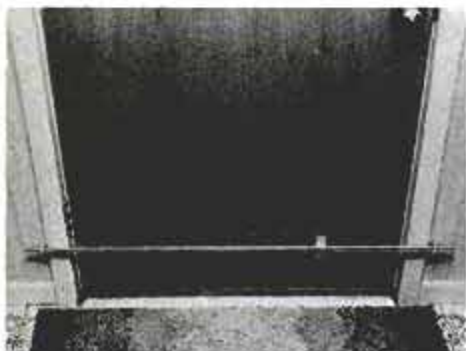
Two hefty screw eyes and a 1/4-in.-dia. by 48-in. steel rod make a simple keyless lock. Wood block spacer holds door shut.
