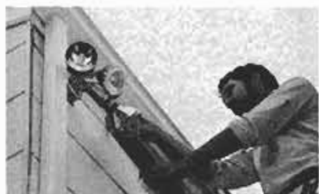
Install floodlights high up, where bulbs cannot be easily removed by an intruder.
