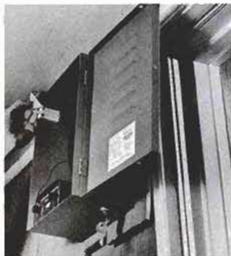
Remove masking tape from plunger switch before closing and securing door of alarm-control box. Switch sounds alarm if door is pried open while system is armed.
