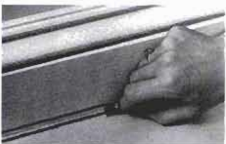
1 Run a crayon or chalk line around the room's perimeter; mark floor and wall.
