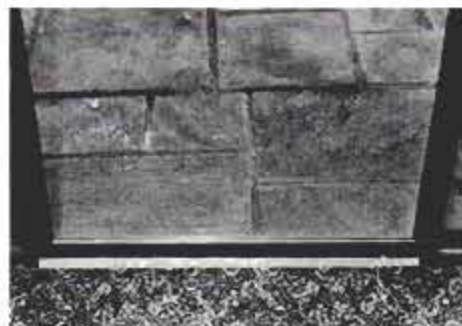
Cut a 1-in.-dia. wood dowel or aluminum pipe to length and place it in the channel to secure a sliding glass door. Tie a string around this lock for easy removal.
