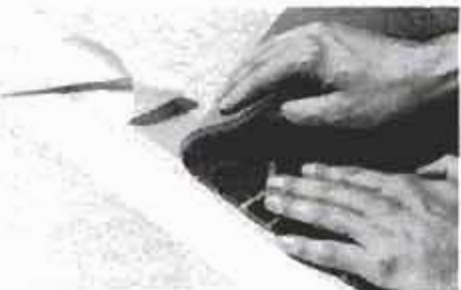
4 Use double-face tape at seams and doors to ensure that the carpet stays flat.
