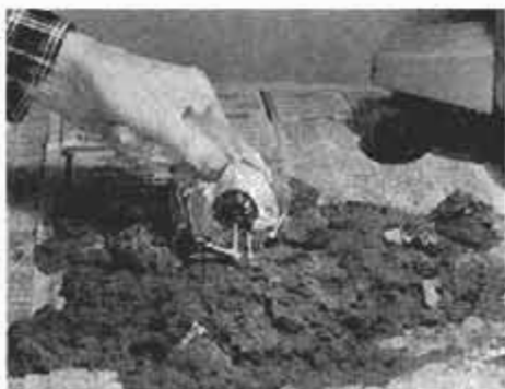
2 Wrap a horseshoe magnet in a plastic bag and search sweepings for missing small metal objects. The plastic keeps the magnet free of metallic dust and debris.
