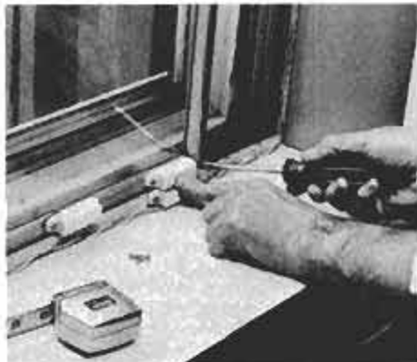
Attach second unwired detector to a window so it can be protected while open for ventilation. It is also a good idea to lock the window in the open position.
