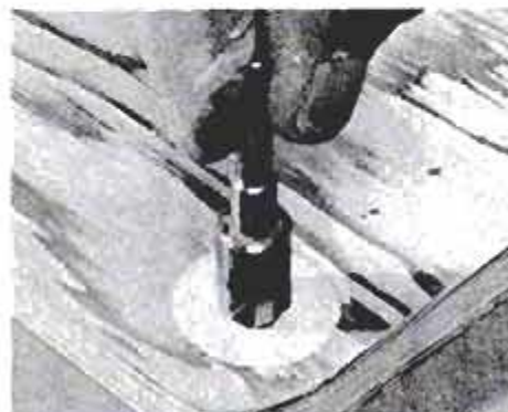
Before filler sets, remove screws. When dry, sand filler flush, then hand-twist a countersink bit to bevel edges slightly.
