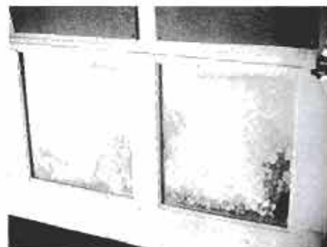
Unsightly mildew like this on single panels will be eliminated because moisture won't condense on insulated double panels.
