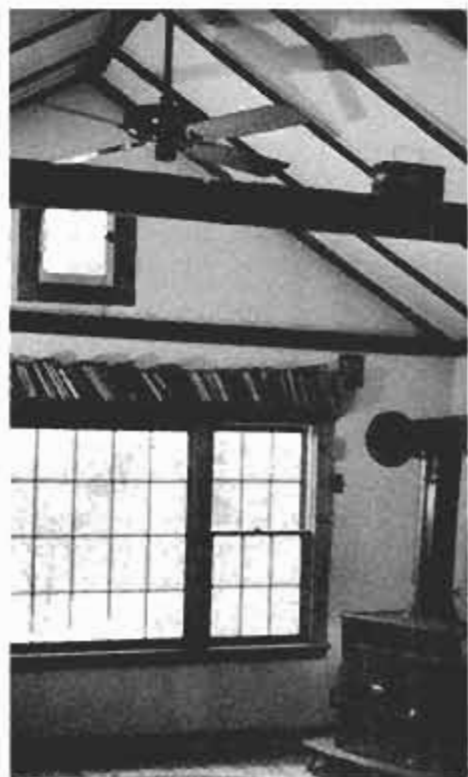
The ideal fan height from the floor is 10 to 12 ft. Switches are to right of window. Heat from the stove also activates fan and thereby contributes more to fuel savings.
