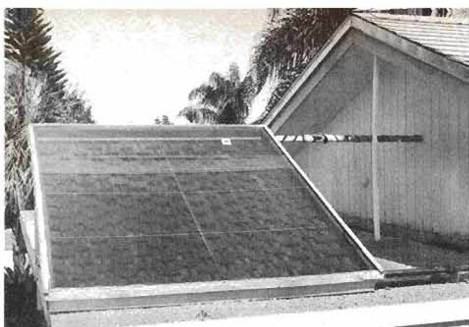
This solar water heater can supply at least 42 gallons of hot water on sunny days. Any handy person who can make good soldering joints on copper pipe can construct it.
