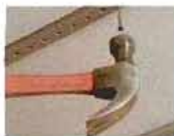
1. Nail up tracks.
