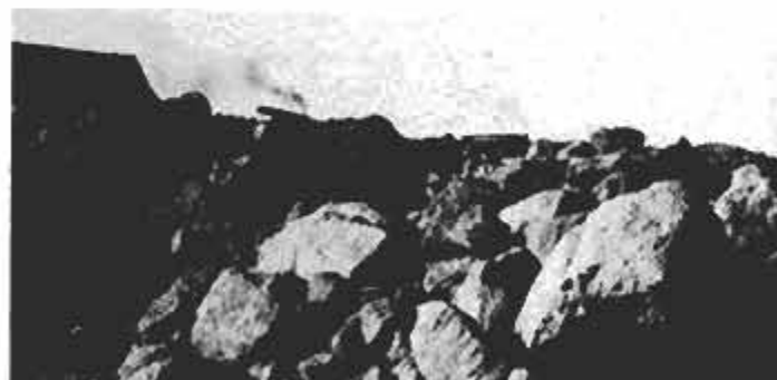
Japanese-made bulldozers are dwarfed by heaps of volcanic rock called tuff. Dozers are solidly built, but too low powered to rip the rock without extensive use of explosives.
