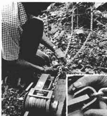
Before use, chain is fastened to winch clevis (Inset) and secured to a tree.
