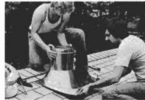
Gently lift roof shingles on upper side and slip the chimney flashing under shingles, as shown. Do not damage other shingles.
