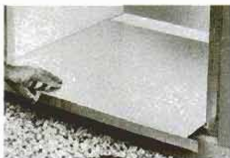
Cut ears of floor sheet as shown in drawing. Install with aluminum nails driven through front edge and into plywood floor behind.
