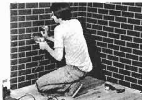
After carpeting is removed, wall panels are placed in intended final position and holes are bored through for toggle bolts.
