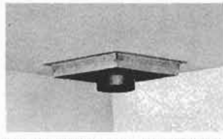
Section of telescopic stovepipe has been placed in the chimney support box. This section allows for final flue adjustment, made by pulling down the lower section.
