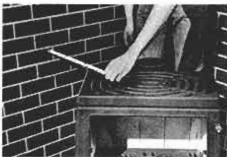
Measure from panel to nearest point on the stove to position stove for minimum clearance allowed by your local building code.
