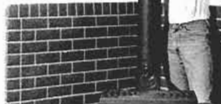
Section of telescopic stovepipe has been placed in the chimney support box. This section allows for final flue adjustment, made by pulling down the lower section.
