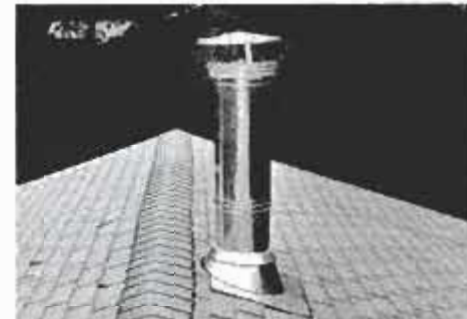
The installation is completed with the chimney cap. According to most codes, cap should be at least 24 in. above roof.
