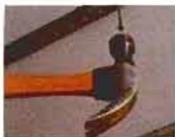
1. Nail up tracks.
