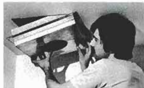
Place chimney support box in position from below and secure by nailing through joists, or headers, if necessary, in the attic.
