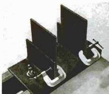
The vise holds three steel parts ready to be tack-welded into a U-shaped channel. The two channel sides are held to the vise jaws with C-clamps. The bottom rests on the side rails, perpendicular to the sides.
