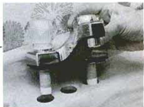
Wrap Teflon tape around threaded shanks before positioning faucet on sink deck. Apply silicone sealant to the underside of the faucet if the sink surface is uneven.
