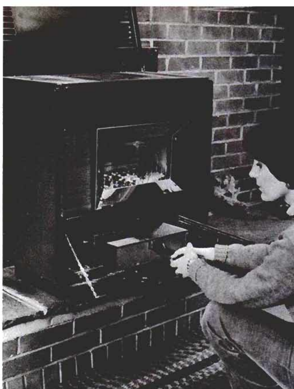
Emptying ash pan assures efficiency. Coal requires more attention than gas or liquid fuels, but less than wood. The model shown is Surdiac No. 508 from Classic Stove Works.
