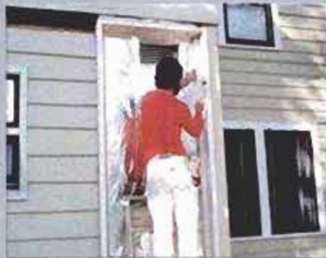
7 Construct the absorber plate frame and install it inside the first frame.
