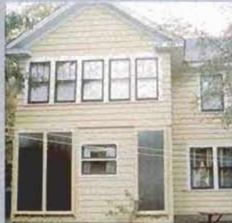
15 Add the batten frame to finish the job.
