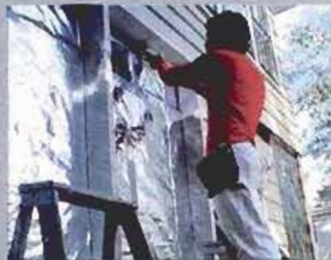
6 To ensure that the frame is airtight, seal up all the joints with silicone caulk.
