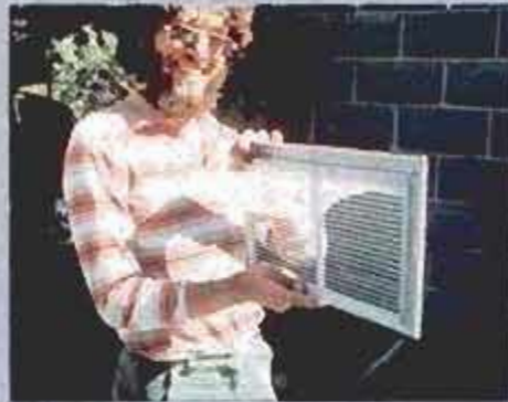
8 The acetate flap duct taped to the bottom vent stops reverse airflow at night.
