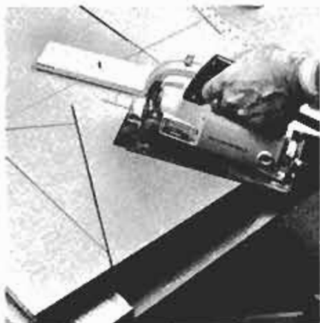
Make the lower, angled cuts of the sidepieces with circular saw and guide strip.
