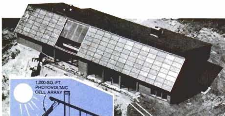
Photovoltaic cells beneath glazed roof panels generate 9,500 kilowatt hours per year—86 percent of total needs for 3,100-square-foot house in Carlisle, Mass.
