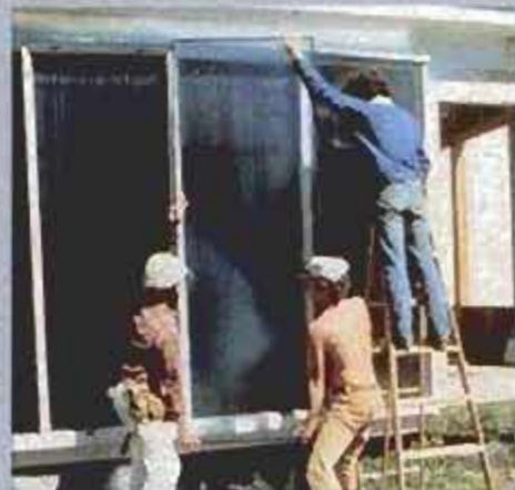
14 Attach the neoprene setting blocks and spacers, position glass and caulk.
