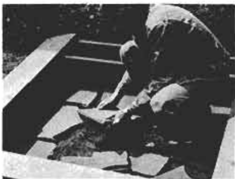
Before adding sand, lay in a slate bottom to prevent soil from mixing with the sand.
