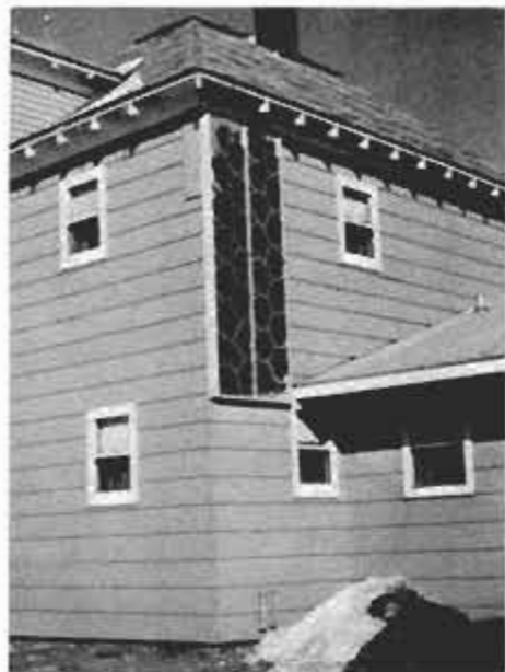
Two-story home has a solar panel mounted vertically at the second-story level to provide supplemental heat from the sun.
