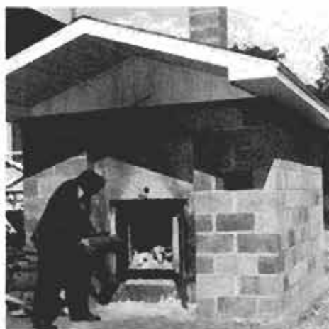
Outdoor furnace, fueled by wood or combustible trash, can heat home and provide domestic hot water all year round.
