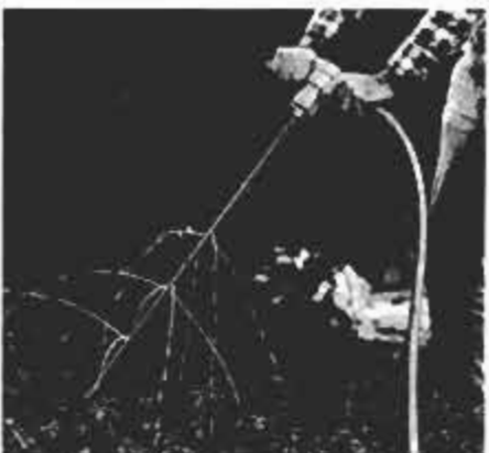
For thoroughness, apply insecticide to surface after injections are completed.
