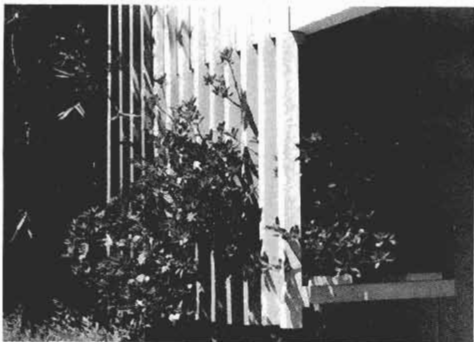
Another way to shade a window—yet allow air to enter and leave the house—is with a sun grille. It's made of 2x3s that are notched and added to an existing roof overhang.
