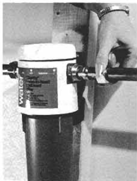
Slip a nut over the pipe and put pipe in the joint opening. This system eliminates need to thread the pipe after cutting it.
