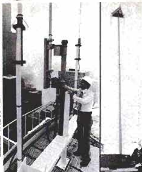
Transmitting and receiving towers for the Advanced Mobile Phone Service (AMPS) are shown above. Photos were taken in the test city, Chicago. There are three towers per hexagonal cell (left), and each tower can relay a message from one cell to another.
