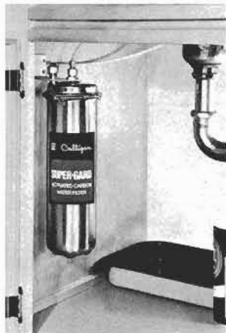
The under-sink taste-and-odor filter by Culligan mounts on a bracket and delivers fresh water to its own water spout. The handy unit is packed heavily with carbon.
