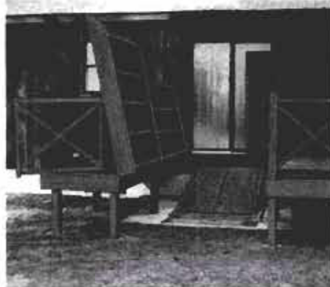
Deck is a good place to entertain. Section C is hooked to the house to prohibit deck access when it's open (above). Sections B and A lift, then are secured to house and rail post, respectively (right).
