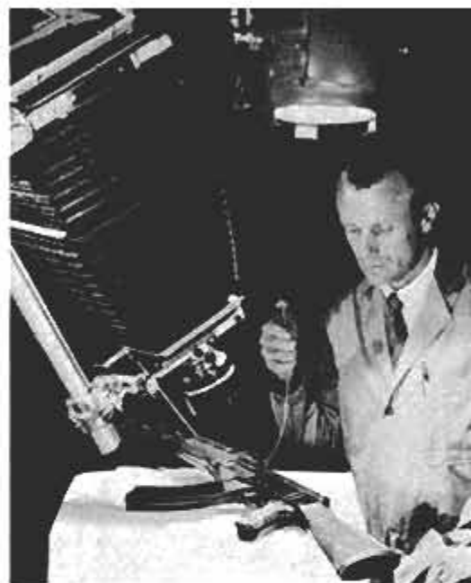
FBI metallurgists use acid to restore filed-off serial numbers on guns used in crimes; numbers are then recorded on film.
