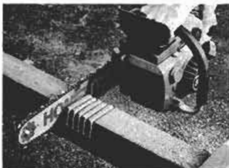
Make inside notches 1¼-in. deep with repeated saw-kerf cuts spaced ¼ in. apart.
