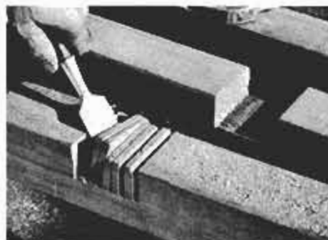
Use wide chisel to remove waste, straighten edges and level bottom of the notch.
