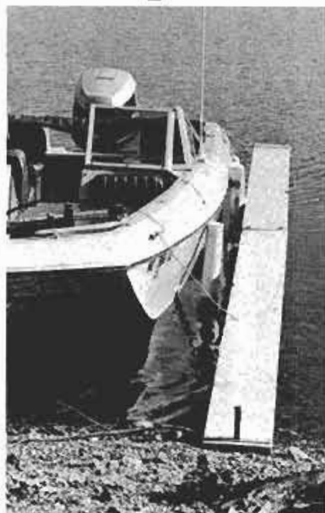
Dock is in position alongside the boat. Bumpers are used between boat and dock.
