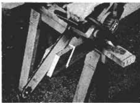
Hold saw at downward angle and rip slowly. Taking extra time now will pay off later.
