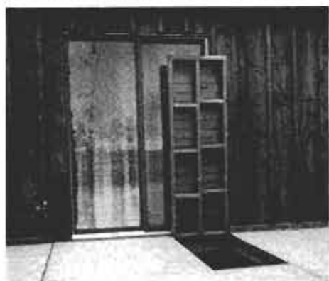
Deck is a good place to entertain. Section C is hooked to the house to prohibit deck access when it's open (above). Sections B and A lift, then are secured to house and rail post, respectively (right).
