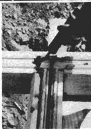
Corner joint shows a double tongue-and-groove log construction. Polyfoam insulation strip and caulking that's applied with a gun combine to create the airtight walls.
