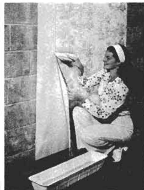
Wall Cover gives smooth surface to cement block and other rough walls. Then you can cover walls with paint or wallpaper.
