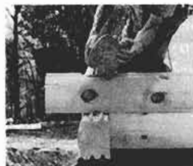
Corner joint shows a double tongue-and-groove log construction. Polyfoam insulation strip and caulking that's applied with a gun combine to create the airtight walls.
