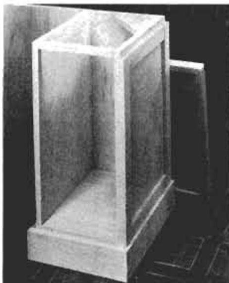
Desk-return detail above shows storage area. Desk frame is being assembled at right. Prebore holes and test fit parts.
