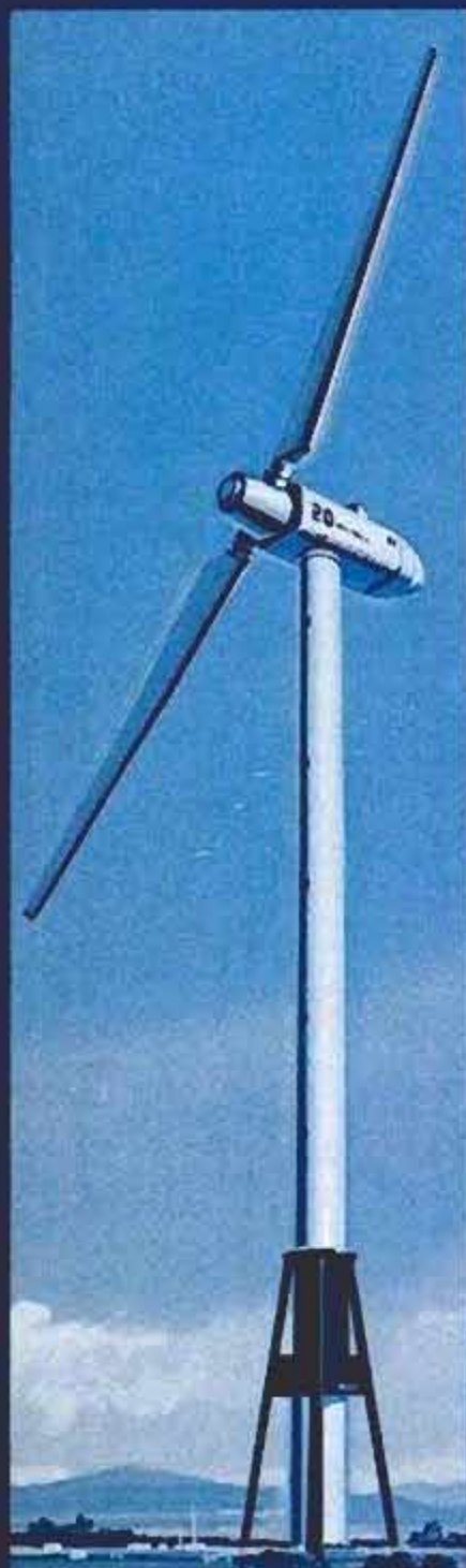
Nacelle's faired end faces the wind as it swivels 260 feet above the ground.
