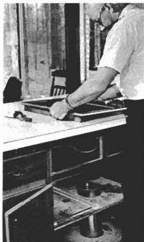
When ductwork is positioned, the grill can be lowered into it and attached. Secure joints with at least four sheet-metal screws, staggered on both sides of joint.
