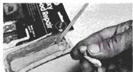
Knead equal parts of the two components to a uniform color. The repair is nontoxic.
