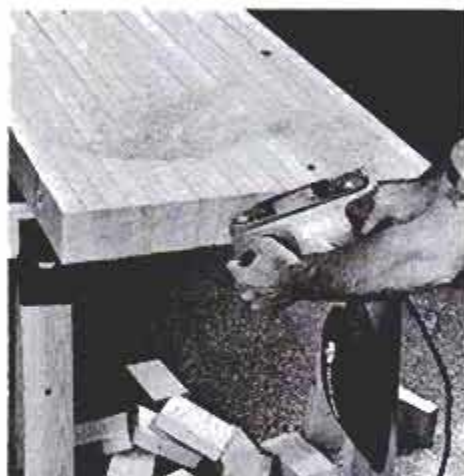
Use a belt sander on the edges. Assemble the top carefully so it won't need sanding.
