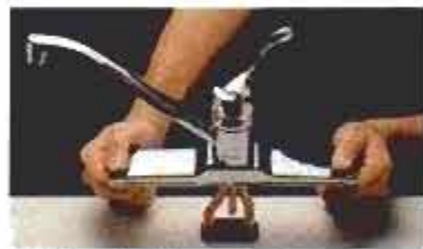
1. All you do is insert the faucet into the deck...
