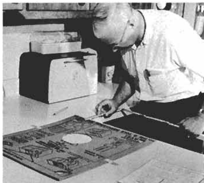
Using manufacturer-supplied template, mark the countertop for grill location. Because the unit eliminates the need for an exhaust hood, it can be placed just about anywhere you want it.
