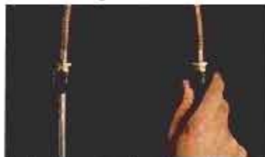
3. Push supply tubes into quick-connectors, tighten the coupling nuts. All by hand. Everything is in the package.
