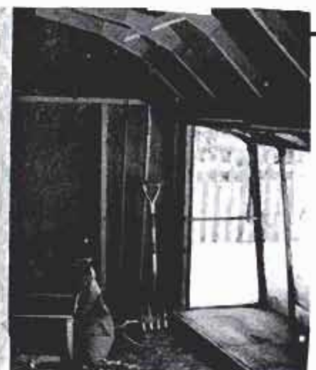
Greenhouse is a simple structure of 1x2 stock covered with hefty plastic sheeting.
