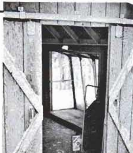
Pair of sliding doors provides an opening big enough to drive a yard tractor through.
