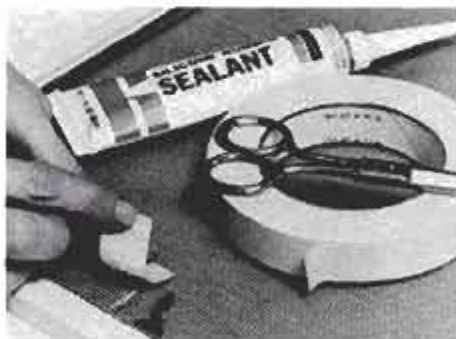
It's no trouble to repair minor tears in metal or fiberglass screening with silicone sealant. First place masking tape on one side of the tear, then apply a thin bead of sealant to the other side. Let cure for 24 hours before peeling away the tape.
