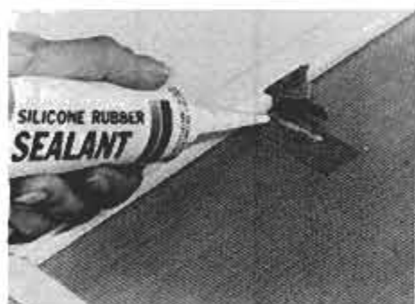
It's no trouble to repair minor tears in metal or fiberglass screening with silicone sealant. First place masking tape on one side of the tear, then apply a thin bead of sealant to the other side. Let cure for 24 hours before peeling away the tape.
