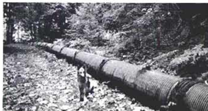
Hydro equipment (above) provides 160 kilowatts to the owners, Susan and John Craft. However, the potential from the stream, which is diverted through a pipe (left), is higher. The Crafts plan to sell excess wattage to others.
