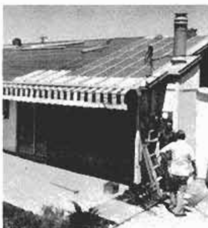
Long house: excess power for sale.
