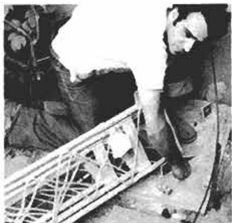
Connecting two out of three bolts will allow the tower to hinge on its base. Four to six people can easily push the tower up.
