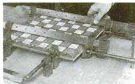
Cut solid edge pieces, mitering corners, and glue them to board. Use four bar clamps, two topside, two underneath.
