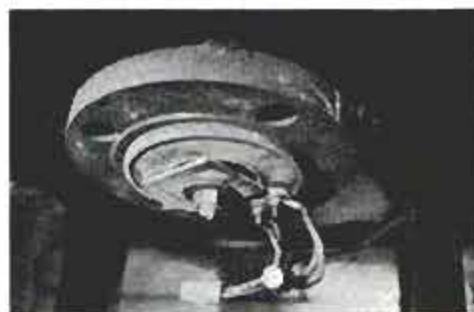
Langhorne attached 450-watt heating element to bottom of a stone coffee table (above and top), which helps heat house.
