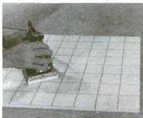
After inlaying strips in perpendicular grooves, sand them flush to playing surface. Use pad sander to avoid gouging.
