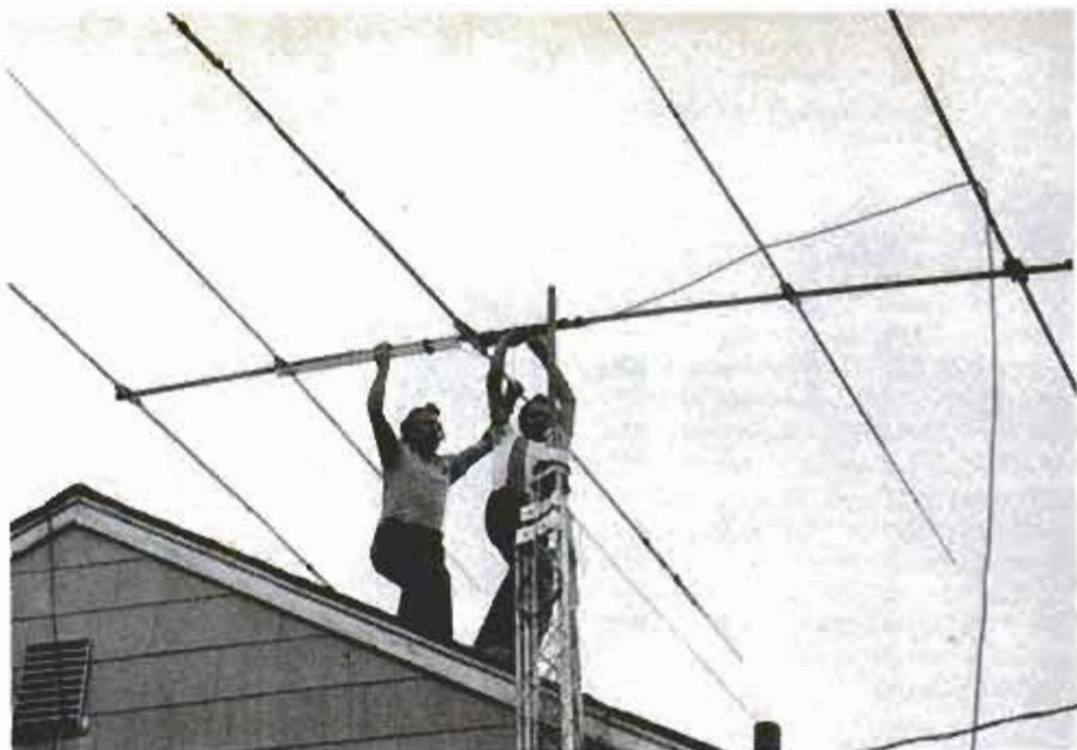
Two helpers positioned antenna mast, but three men would have made the job easier.
