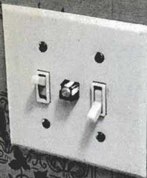
Conserve energy by adding an indicator lamp to a switch that controls an out-of-sight lamp (such as in an attic). It glows when the light is left on.
