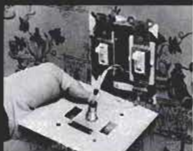
To install an indicator lamp on a multiswitch plate, you need a diode between each switch and the lamp. Twist the diode leads together (inset), solder ends to light terminal (left) and connect them (right) so diodes have same polarity.
