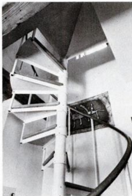
Narrow stairwell connects living room to new bedroom. In summer, air passes from floor to floor through door connecting bedrooms and exits through a skylight.
