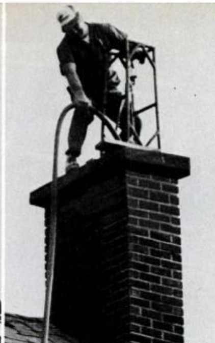
Cement mixture is pumped between bladder and interior wall of chimney.
