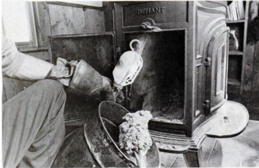
Creosote buildup in the stove acts as an insulator and quickly reduces its efficiency.
