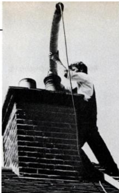
Inflated bladder, inserted in flue, serves as form for cement-lining mixture.
