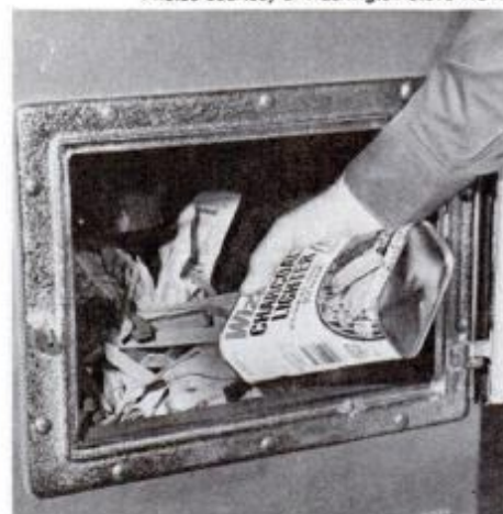
Chemical fire starters are not safe for use and aren't good for the stove, either. The quick temperature rise may ward firebox.
