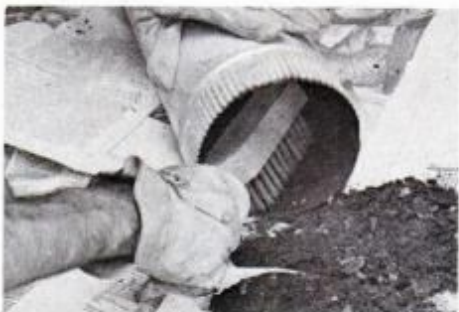
Stovepipe and flue had to be brushed clean at the end of the heating season.
