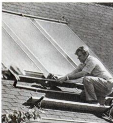
PM's home and shop editor on the roof last year, installing solar-collector plates.
