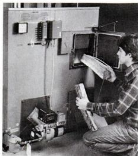
During winter, the boiler firebox walls required a weekly five-minute scraping.
