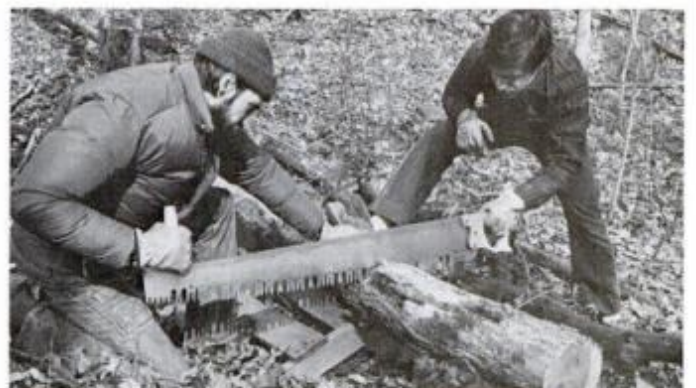
Once tree is on the ground, use sawbuck and one- or two-man buck saw to cut log into desired lengths. Remove bark at cut.
