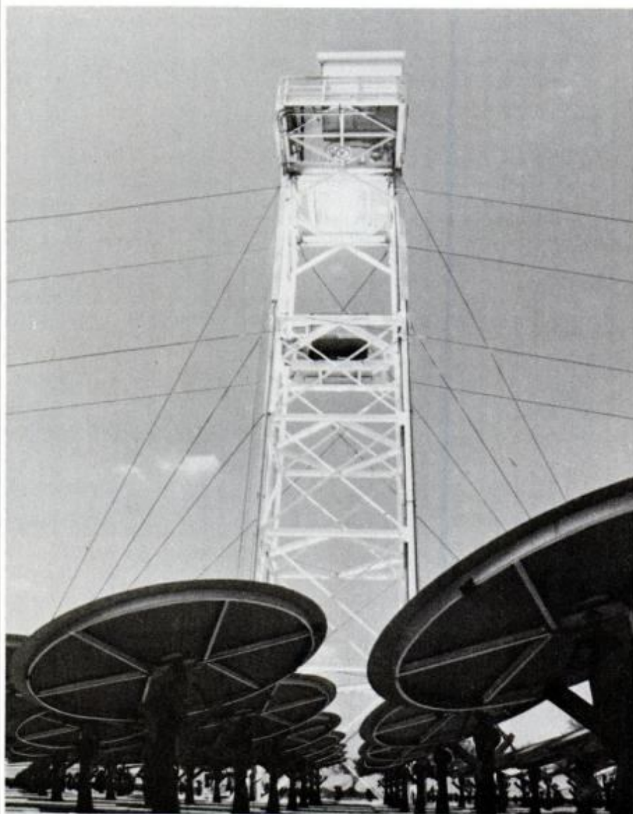
A field of 550 mirrors can raise temperatures at a focal zone to 3500° F.
