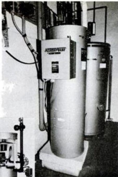
In Hydro-Pulse heating unit (above and left), air and gas are mixed in a sealed chamber and a sparkplug ignites mixture. Hot gases are forced through heat exchanger that's surrounded by boiler water (below).
