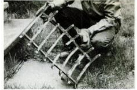
Here's what the ravages of a hot ember fire can do to cast metal. The middle support is missing; others are corroded.
