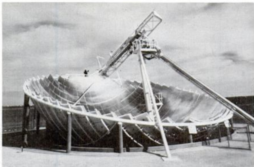
A 65-foot-diameter bowl focuses sun to heat water-filled tube at focus.
