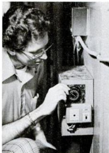
Enertrol model, suitable for boilers with tankless coils, allows you to program for periods of high domestic hot-water use.
