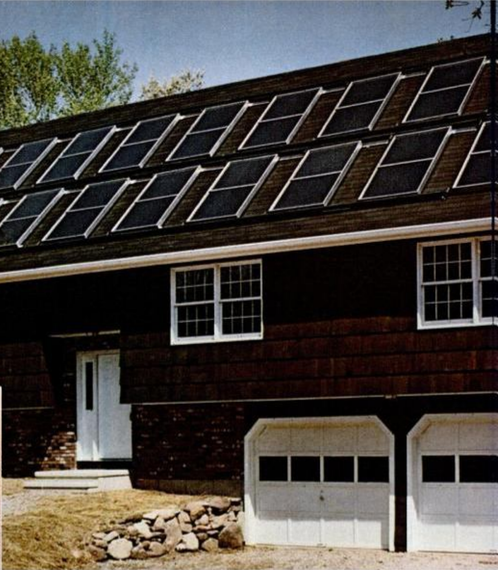
Most of the windows face south to maximize direct solar heat gain. Eave is sized so projection shades windows during warm months. Note shadow line at noon in early May.
