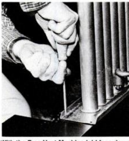
With the Free Heat Machine laid face down on the floor, the tube assembly is attached using screws into the predrilled holes.
