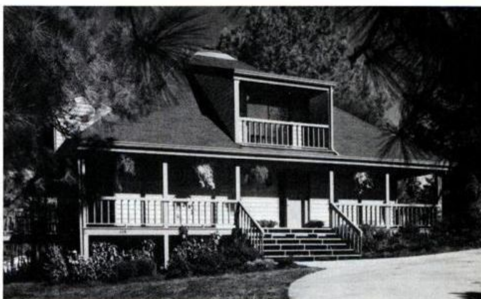
Roof overhang shelters veranda and shades windows and doors from hot summer sun.
