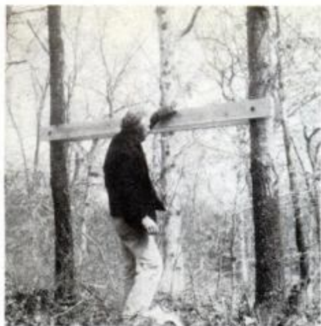
To level beams, secure one end with lagscrew and swing board up until level. Mark tree, secure second end with lagscrew.
