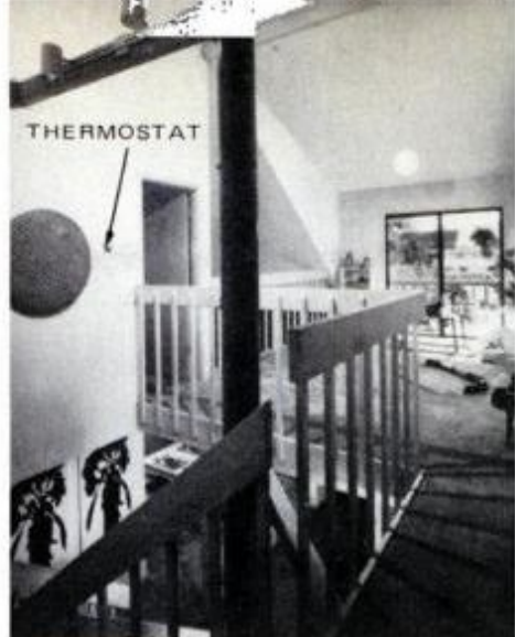
Thermostat in loft area activates the blower when temperature reaches a preset limit.
