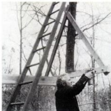
To level beams, secure one end with lagscrew and swing board up until level. Mark tree, secure second end with lagscrew.
