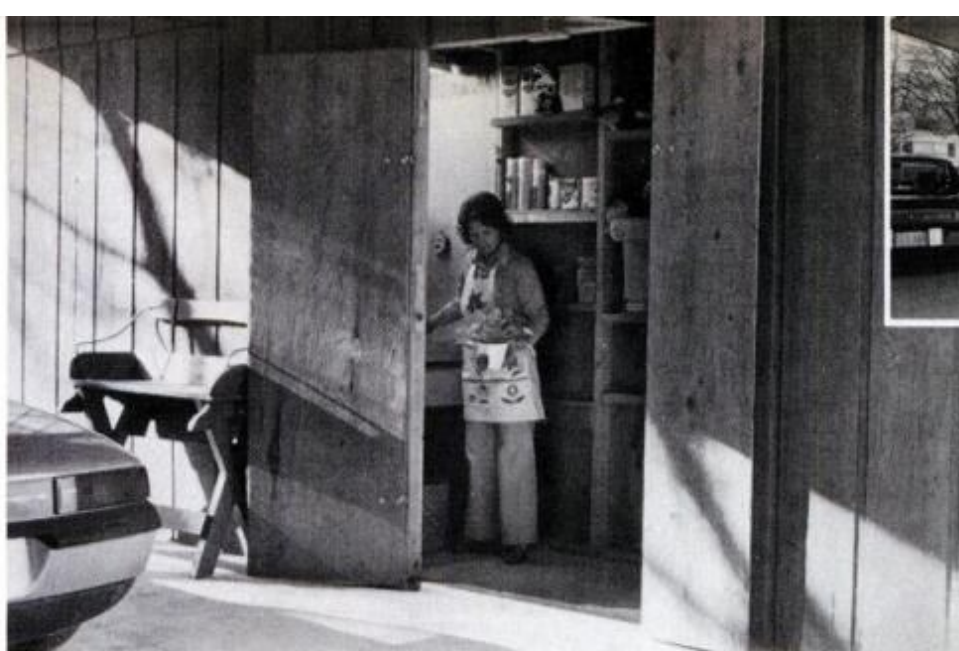
The 3-ft.-wide storage area, which forms outside wall of carport, holds bench.
