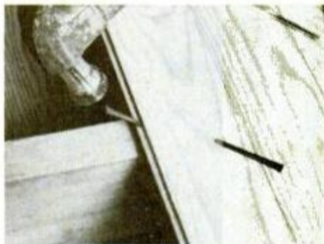
Blunt-pointed, cut flooring nails minimize splits in flooring tongues. Use a blunt nailset to set all nailheads flush.
