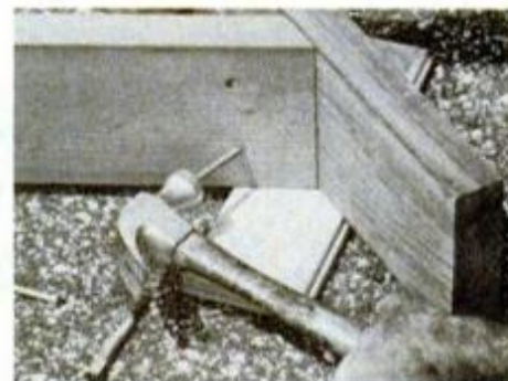
Choose hot-dipped, galvanized common nails for outdoor wood construction to prevent the corroding effect of the weather.
