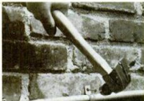
Drive hardened masonry nails into mortar joint using at least a 20-oz. hammer or a hand mallet. Since these nails chip and break easily, wear your safety goggles.
