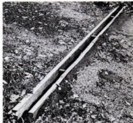
Shop-built driveway channel eliminates flooding of the driveway at its low end.
