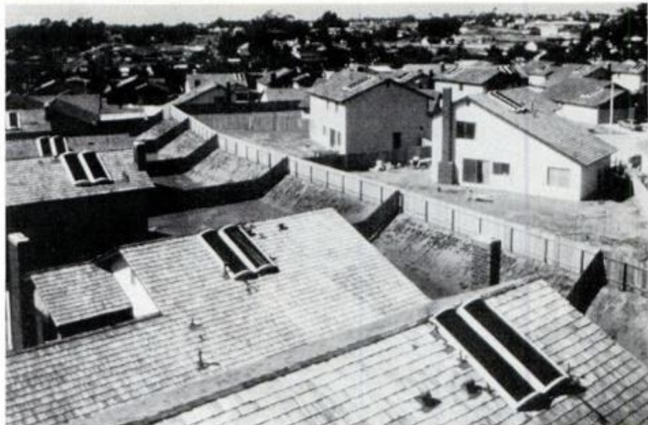
What’s wrong with the picture above? Haphazard orientation of collectors reduces efficiency. Ideally, collectors should face no more than 15° east or west of true south. Moldings lifting on collector surface (below) is evidence of poor construction.
