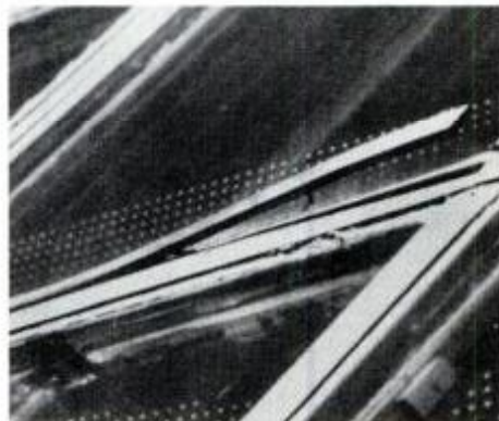
What’s wrong with the picture above? Haphazard orientation of collectors reduces efficiency. Ideally, collectors should face no more than 15° east or west of true south. Moldings lifting on collector surface (below) is evidence of poor construction.
