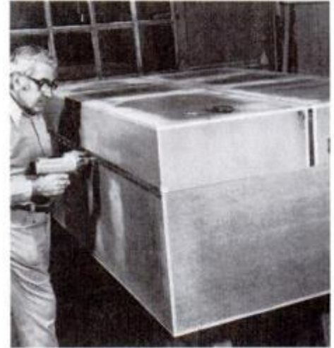
With the doors resting in place on the cabinet, attach the hinges. Shims are used to create a small gap at the hinge edges.
