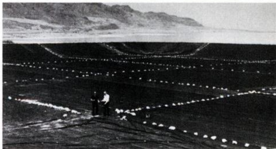
Shallow pond, shown before filling with Dead Sea water, collects heat near briny bottom.
