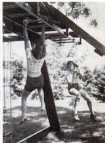
Hand-over-hand climber was made from a discarded wood ladder with round rungs.
