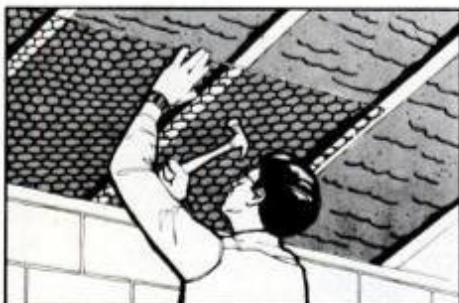
Wire mesh secures underfloor insulation.
