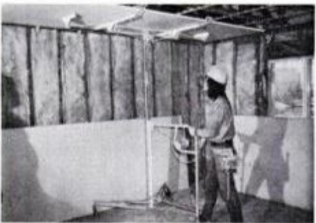
This lifter makes it just as easy to install a drywall panel above the waist level (above) and on ceiling (below).
