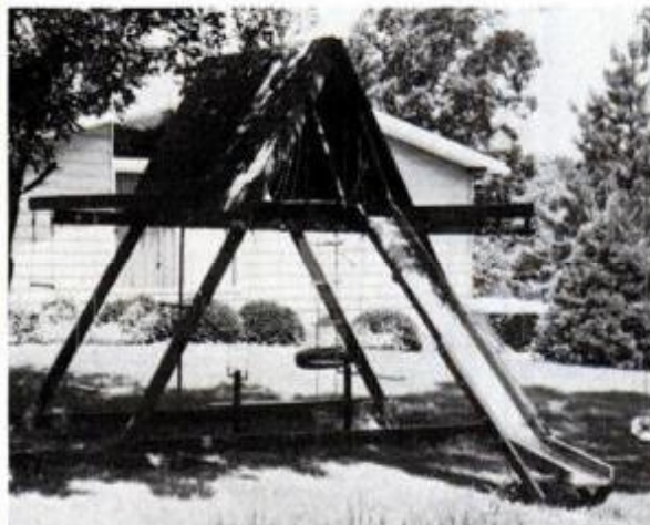
Opposite view shows sliding board made of heavy-gauge, galvanized sheet metal.
