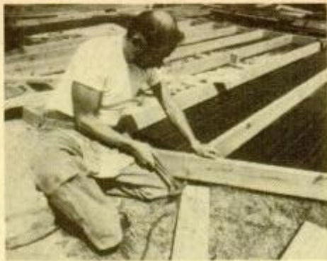
Lower-level joists are fastened with two 16d galvanized common nails spiked through header joists. Use slate or pressure-treated wood as shims if needed.
