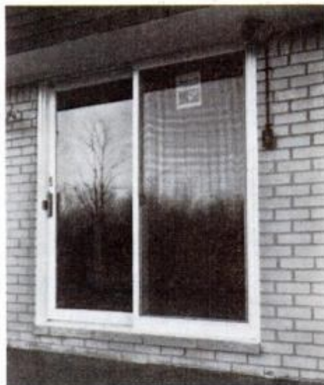
This sliding wood door fits in the same size opening as most 6-ft. sliding metal doors.
