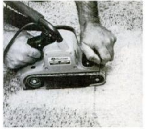
Use a belt sander to remove final traces of wax and to roughen floorcovering's surface to provide tooth for mastic.
