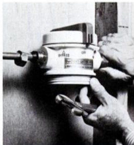
Engage locknuts by hand; then tighten with a wrench to make watertight seals.
