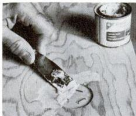
Partially driven staples can effectively serve as key that will help to lock wood filler in a shallow patch.
