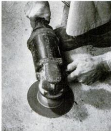
When installing a floor directly over concrete, first level off the high spots with a heavy-duty disc sander or surfer.
