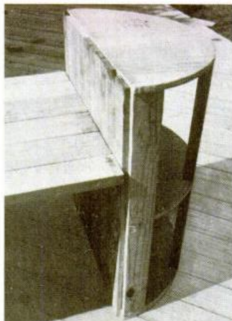
Cleat supporting tabletop is fastened to counter to put dining table at 30 in. height. Use 1x3 boards for the tabletop, leaving a slight gap between the boards.
