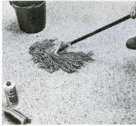
Mop with wax-remover solution to clean wax from resilient flooring. Scrub brush may be required on spots thick with wax.
