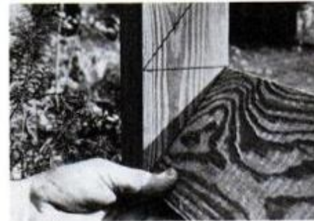
Board's edges are lined up with the pencil mark on post edges as shown.
