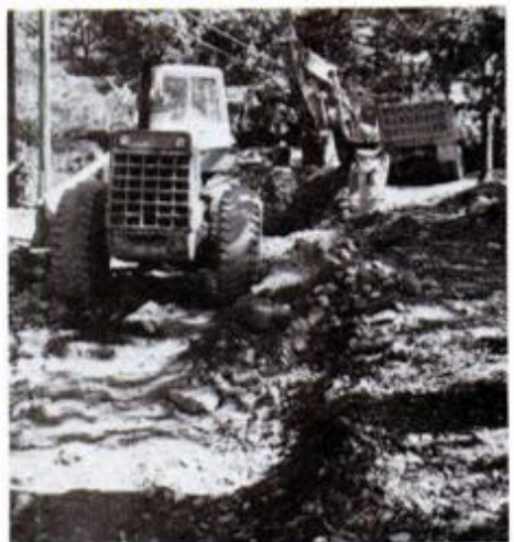
Municipal road-widening and sewer projects leave many cords of wood behind.
