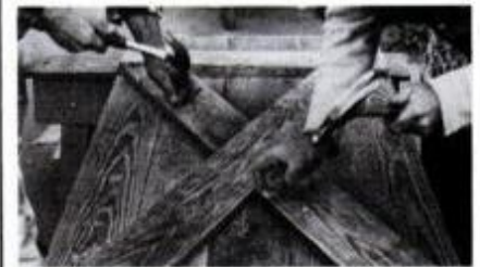
X-brace adds strength and a rustic look. Boards can be butted or lap-joined.
