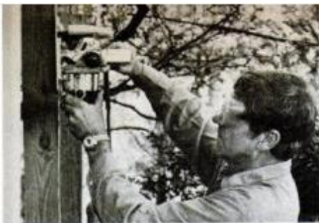
In some cases, it is easier to install a post, then mark and cut it off in place.
