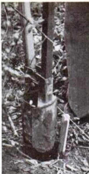
Clamshell posthole digger gives neat holes for more rigid post installation.
