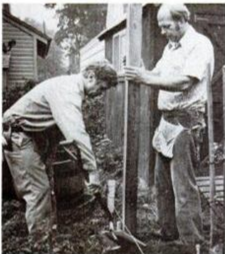
It's easy to set post when one holds it plumb while second backfills and tamps.
