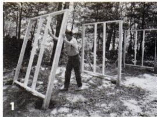
1 Side and center walls are framed on ground, then tilted in place and braced, so concrete collars can be poured.
