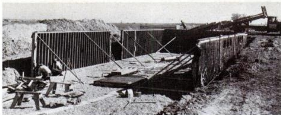
All-Weather Wood Foundation is constructed of pressure-treated lumber and plywood. The concrete slab is poured last to cover wood sills and anchor the wall studs.
