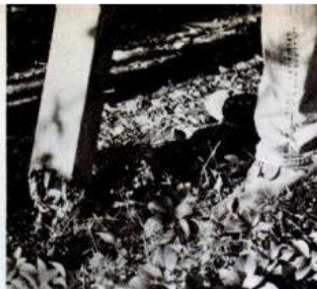
Non-pressure-treated posts failed because of rot below grade, reducing the 11-year-old fence at right to fireplace kindling.
