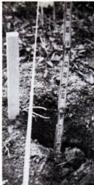
On the fence shown, holes were dug to about 18-in. depth; note marker stake.
