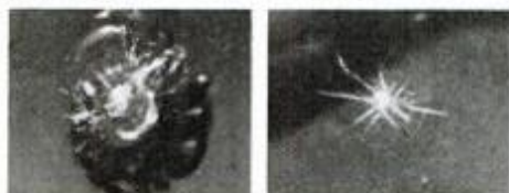
Top: When plunger is up, vacuum draws air out of solution in pedestal. Above left: "bull's-eye" crack before repair. Above right: After, it's resin-filled, hard to see.
