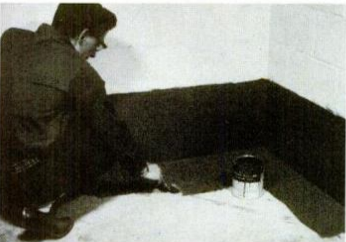
Spread two-part epoxy sealer with a polyester brush. Do not mix more than you can handle—or compound will begin to set.
