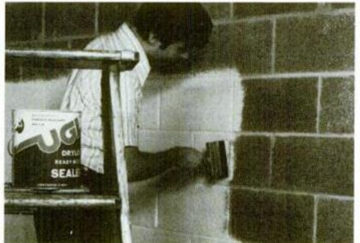
Apply single-coat, Portland-cement-type sealers with a stiff brush to get the granules into masonry pores.
