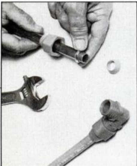
Slip a plastic nut (Qest is shown) over copper tubing; then slip on metal ring.
