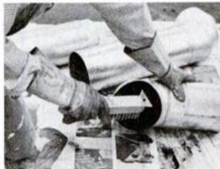
Don't neglect dirty stove pipes either; 1/4-in.-thick encrustations should be scrubbed clean before cleaning stove.
