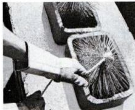
Flue can also be scrubbed by tying rope to both ends of brush, stationing helper below and alternating pulls on ropes.
