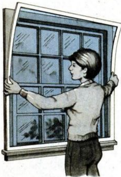
Easy-to-assemble inside storm window fits over window-frame casing for extra protection during winter power outages.
