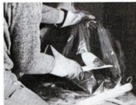
Carefully scoop creosote from smoke shelf into trash bag. If you don't own an ash shovel, use a child's sand shovel.
