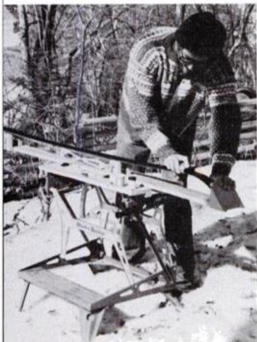
Waxing bench holds ski firmly so that tip may be cleaned, waxed and smoothed.
