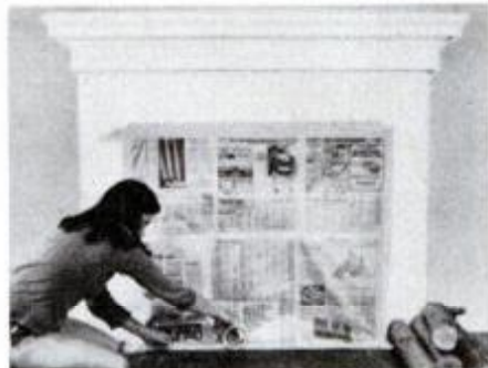
As precaution against airborne soot, tape old sheet or newspapers to fireplace opening before scrubbing from roof.
