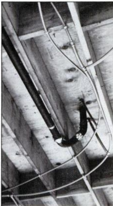
When flexible PB tubing is used, corners can be negotiated without elbows or tees.
