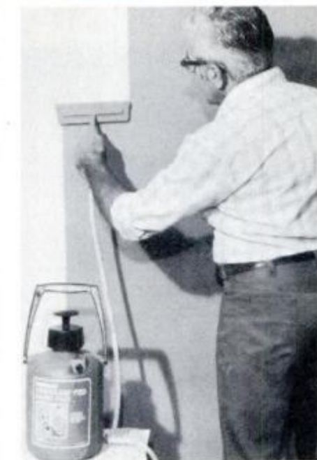
Hand-pressurized painting unit, made for water-soluble paint, lets you work without constantly reloading the applicator.
