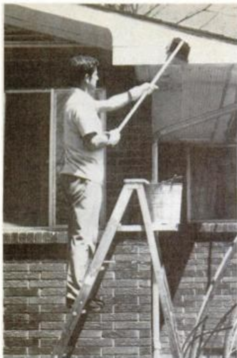
Before repainting a house, use a long-handled brush and hot lye to strip old paint.
