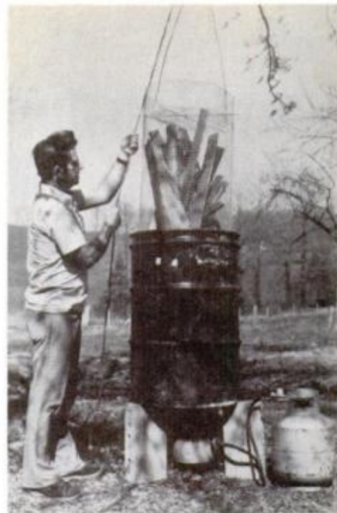
A lye-dipping tank makes easy work of stripping used lumber and furniture.
