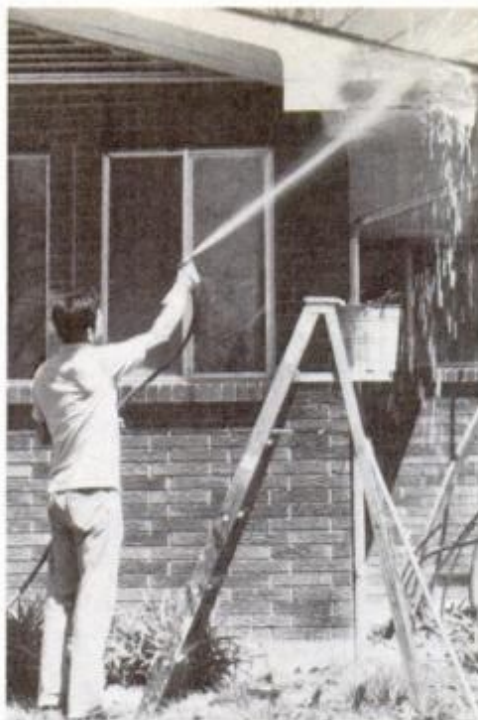
Softened paint hoses right off to expose wood. Scrub with weak acid to neutralize.
