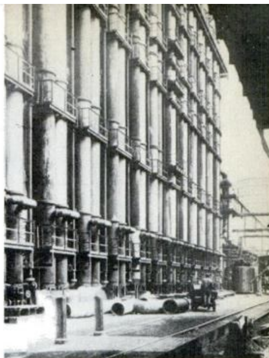
This is the bank of reactors for treating coal to get quantities of synthetic crude oil.
