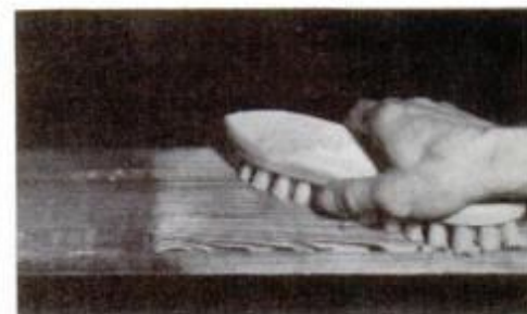
Brush on full-strength laundry bleach to restore the wood to its natural color.
