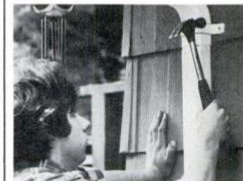
Downspouts are conventionally installed with galvanized nails securing straps.
