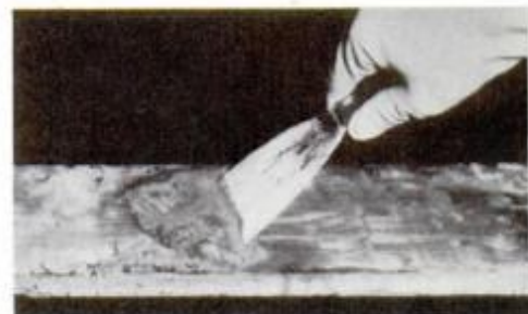
Layers of tough, hard paint seem to melt under the action of a hot lye solution.
