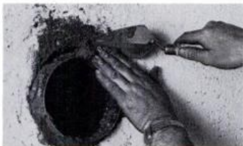
Before flue pipe was passed through wall, thimble was mortared in place. Then flue pipe was inserted and the joint sealed.
