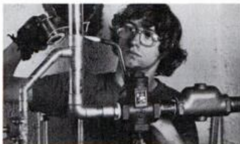
Air purger, valves and copper pipes were plumbed and soldered according to the manufacturer's recommendations.
