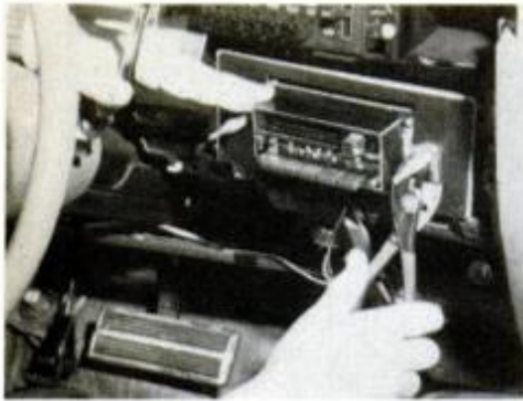
Make sure that the radio works before finally securing it into the dash. Then tighten the nuts on the two shafts that secure the radio to the mounting plate.
