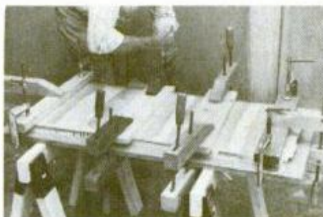
Strip assembly is then glued to plywood (J). Use wax paper between clamping blocks and work to prevent accidental bonding.
