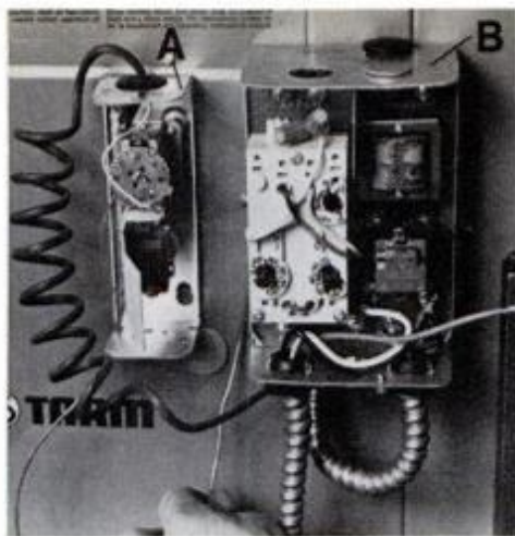
Connecting overheated control (A) and master hot-water control (B) normally requires skill of a professional.
