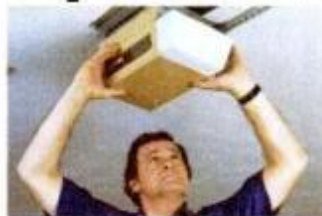
Attach power unit to ceiling
