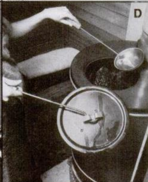
A Double-glazed roof, windows on solar greenhouse help to retain the heat. B Roof vents permit excess heat to escape on warm days (also see drawing). C Water-filled tubes are heat bank. D Excess heat from wood-burning sauna stove supplements solar heat gain. E Cattle trough is additional heat bank. It also functions as a hot tub.
