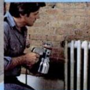
Paint Radiators and Pipes
