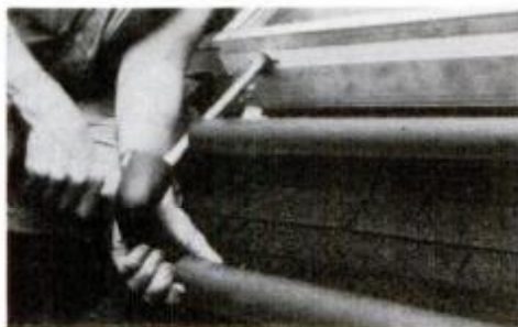
Armaflex wrapped around elbows and taped prevents heat loss at these points, too.
