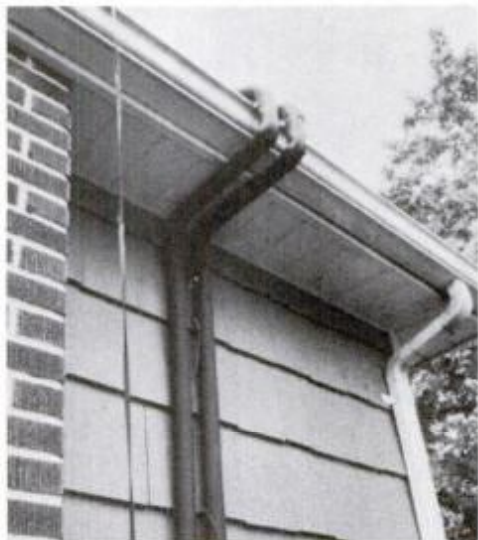
Pipe elbows around gutters. Straight run requires holes through cornice.
