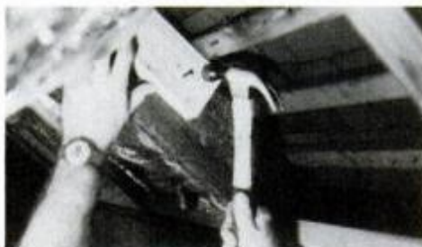
Use 16d nails to secure the cat. See art on page 135 for the blocking technique.
