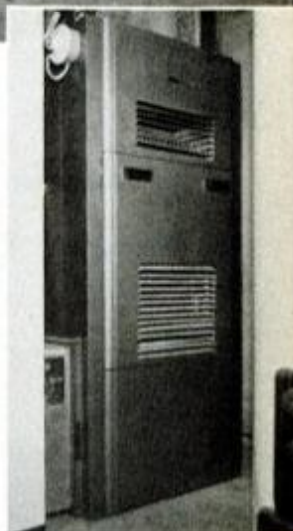
Space between the new furnace and the old furnace cabinet is filled with fireproof insulation (above). At right, the furnace installation is complete and the front panel is in position. An exploded view (below) shows old furnace cabinet with new furnace replacement. A plenum adapter was made to fit plenum opening of new furnace to existing hot-air plenum.
