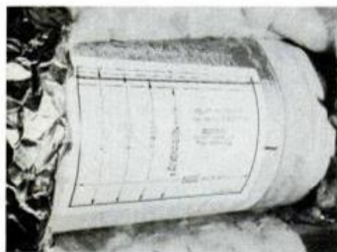
Self-adhesive template in the kit serves as a guide for cutting a hole in the duct.
