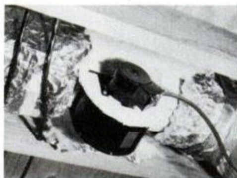
Unit's motor runs at 1550 rpm; it mounts out of the airstream to lengthen its life.
