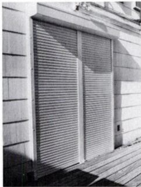
Exterior-mounted rolling shutters cover this 6-ft.-wide sliding glass door between den and deck. Shutters lower heat gain in summer, heat loss in winter, protect glass from hail or sleet, afford full privacy.
