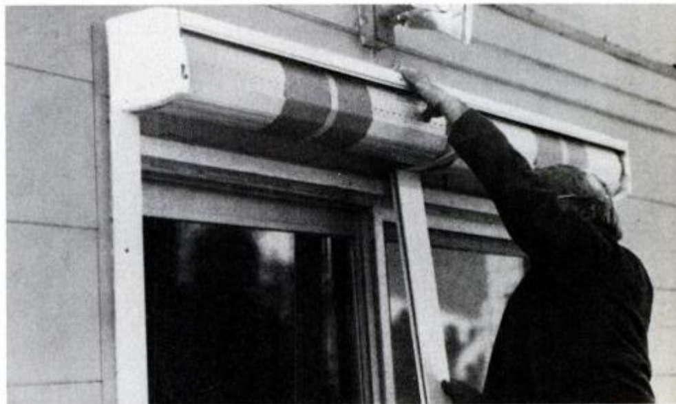
Lift shutter assembly and attach it with screws to the horizontal filler. In the project shown, two shutters separated by a center post are installed.
