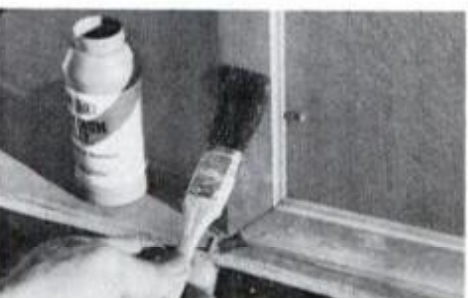
Renew corroded aluminum by applying Aluminum Jelly. The thick gel solution stays put, even on vertical surfaces.
