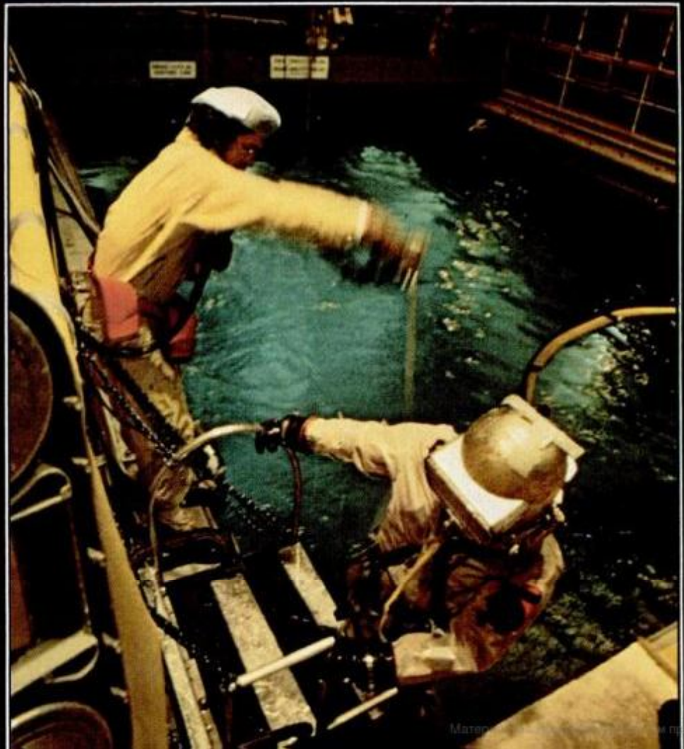
By carefully limiting the amount of exposure to radiation, divers can work safely in nuclear reactor installations, performing inspections or mechanical jobs. Precautions against contamination must be thorough.
