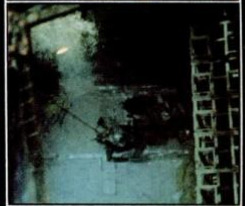
By carefully limiting the amount of exposure to radiation, divers can work safely in nuclear reactor installations, performing inspections or mechanical jobs. Precautions against contamination must be thorough.
