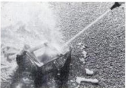
Remove all traces of chemical with thorough water hosing after curing.
