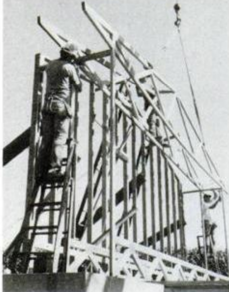
House viewed from end shows truss roof fully in position on wall plates.
