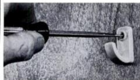
As screw is turned, plug inside expands.
