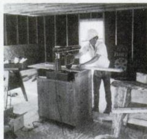
House is quickly framed and sheathed so crew can use interior for work area.
