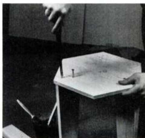
11 Cut plywood seat bottoms and tapered legs and glue and screw the plywood to legs. Countersink screw heads.
