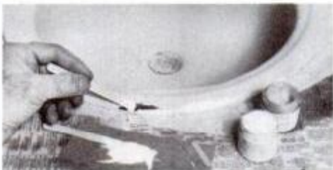
A patch filler builds up chipped areas. It is sanded flush to the adjacent areas.
