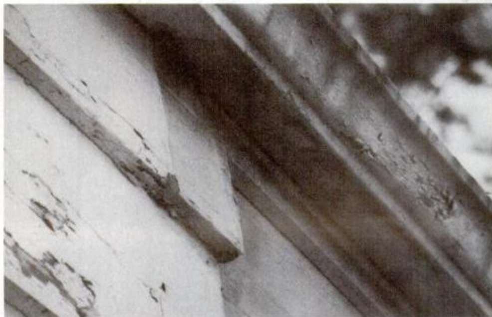
Joints between dissimilar building materials, such as at the doorsill (right), should have been caulked to prevent water infiltration and the consequent paint peeling and rot.
