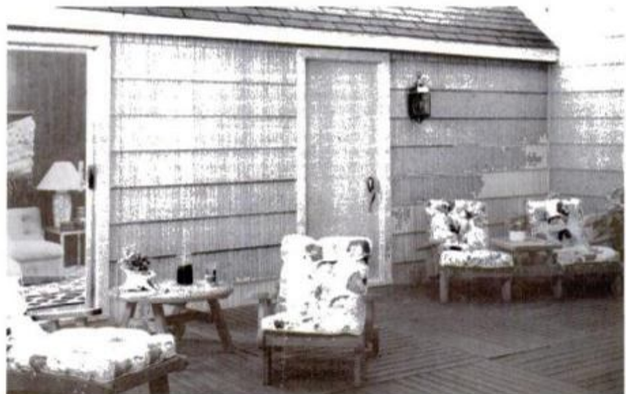
Cedar shingles? No, they're actually horizontal strips of hardboard embossed to look like courses of shingles. "Courses" are available in 16-ft. lengths.
