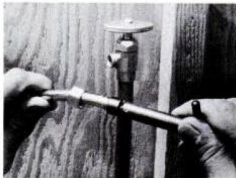
One bead on the tubing seats against the valve fitting, the other against the nut.
