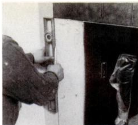
2 Set all tiles over fireplace, draw vertical line for setting tiles below.
