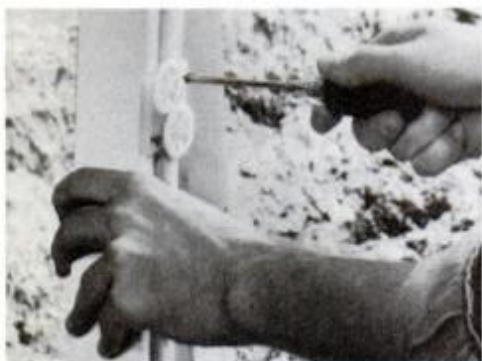
2 Peachtree insulated glass patio doors can be installed to slide left or right depending on the roller placement.
