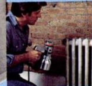
Paint Radiators and Pipes
