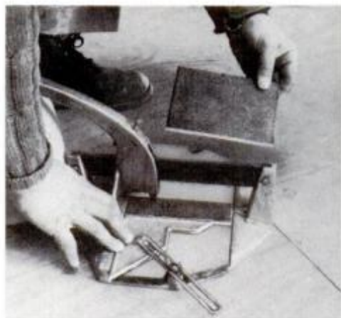
4 Cut border tiles with power saw or with hand-operated cutter (shown).
