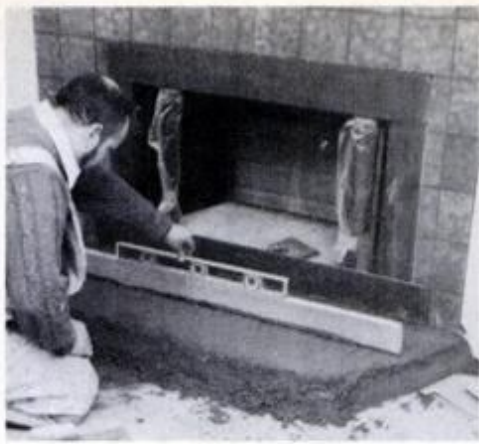
9 Screed mortar bed with a straight board; check with a spirit level.
