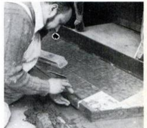
13 Position edge tiles carefully so the joints line up properly.
