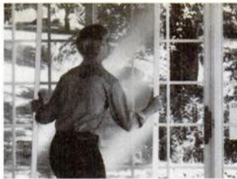
3 Inside screens stay cleaner than conventional screens, and are easily removed in winter to let in solar radiation.
