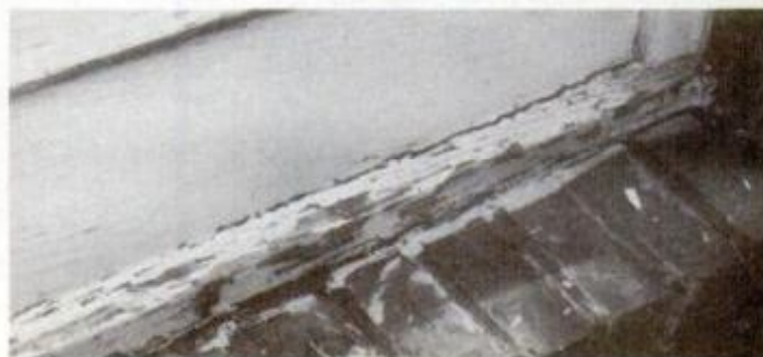
Joints between dissimilar building materials, such as at the doorsill (right), should have been caulked to prevent water infiltration and the consequent paint peeling and rot.
