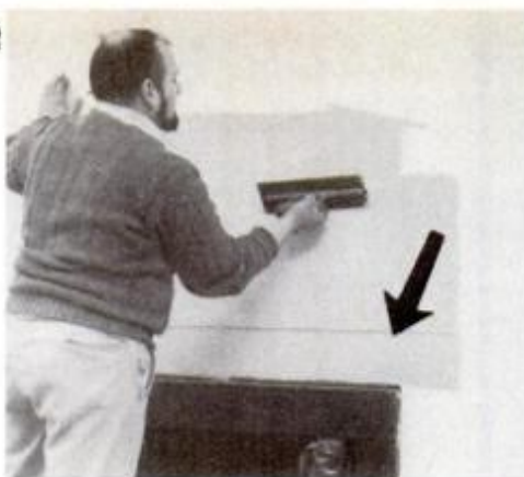
1 Spread wall tile adhesive over drywall. Level line (arrow) guides courses.
