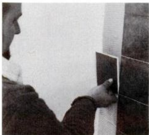
6 Make certain the border tile joints line up with the full tiles.
