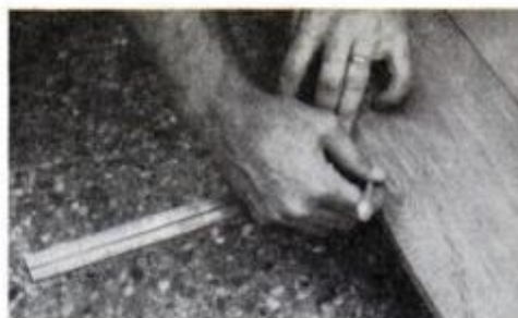
Inside circumference line is accurately drawn \frac{3}{8} in. from edge (at bottom).
