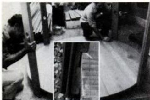
Each stave is tapped with a mallet, so that slot engages, as in inset photo.
