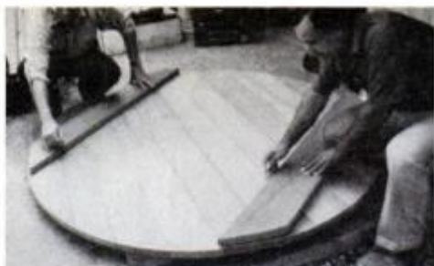
Staves for plumbing connections are located after determining where seats go.
