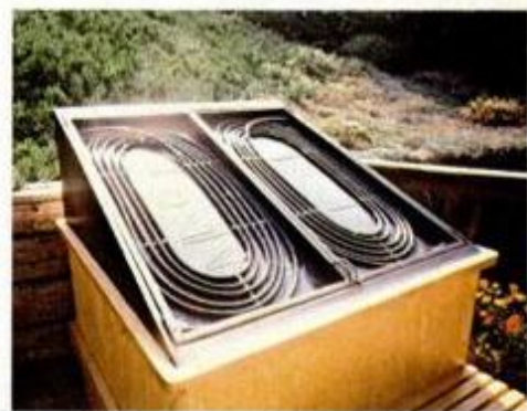
The top-cover doors (left) are framed fitted with clear acrylic and black polyethylene. Black plastic irrigation pipe (above) is sandwiched in between these layers.
