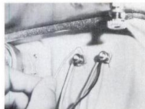
9 To make the electrical connection, fasten prespliced wires to each terminal on unit by tightening thumb nuts.
