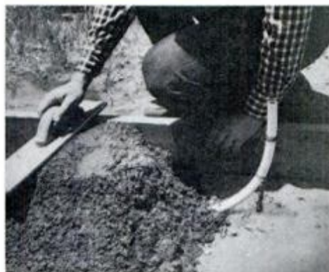
Special pipe hangers hold CPVC snugly (left), but leave play for expansion and contraction. Use at least one hanger every 32 in. PB can be used beneath concrete slab (above). Install joint-free runs, attaching fixtures to exposed pipe ends located above the slab.
