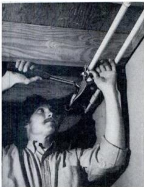
Special pipe hangers hold CPVC snugly (left), but leave play for expansion and contraction. Use at least one hanger every 32 in. PB can be used beneath concrete slab (above). Install joint-free runs, attaching fixtures to exposed pipe ends located above the slab.
