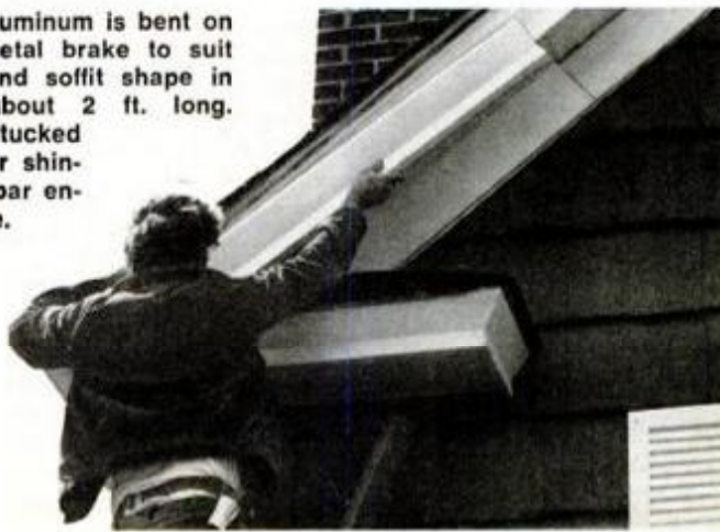
New fascia board (arrow) is installed to provide a solid base for metal cladding.
