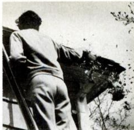
Debris, nest material squirrels hauled in is removed, then attic is vacuumed.
