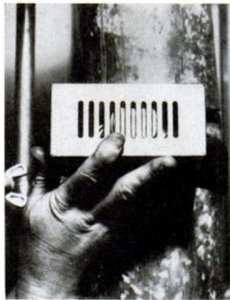
Automatic vent damper is placed between pipe sections. If necessary to fit unit, push upper pipe further into chimney.
