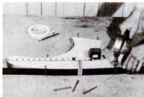
Use 10d common nails into bench top to hold runner for bending steel edge.
