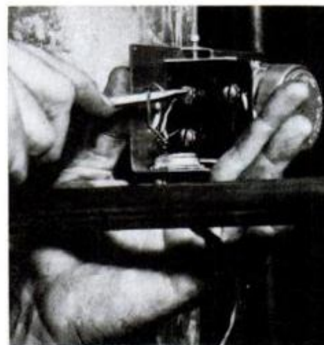
To facilitate installation, terminals on motor (above) are numbered to tally with the time delay terminals.
