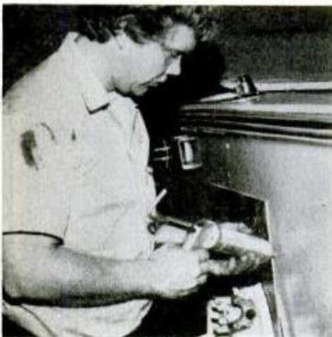
The watertight bond for the new aluminum transom plate was provided by bedding it in place in a silicone sealant.
