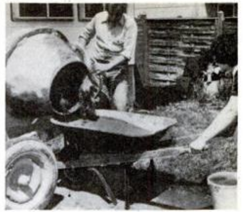
Small rented, gasoline-powered cement mixer saves time and back muscles.
