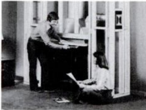
Position the warm air vents on the side. Next, frame out the fireplace with studs.
