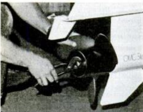
Attachment of outdrive seal, drive unit and finally the exhaust-hub propeller were finishing steps. Transom was then painted.
