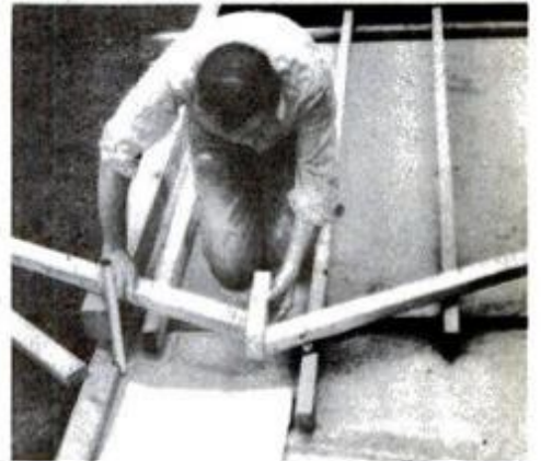
Two-by jig spaces rafters for ridgeboard when you lay out wall.
