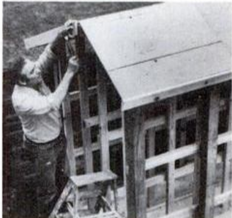
Sheath roof with 3/4-in. exterior grade plywood, then add rake and fascia boards.
