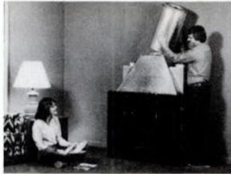
To install this Heatilator easily, site the unit, fasten chimney starter section.
