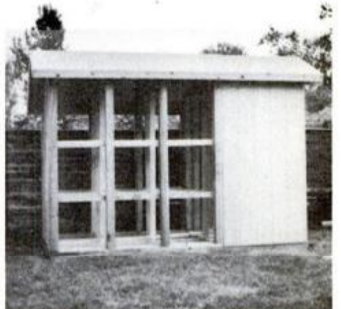
Use a 15-lb. felt under cedar shakes on the roof, T1-11 cedar boards for siding.
