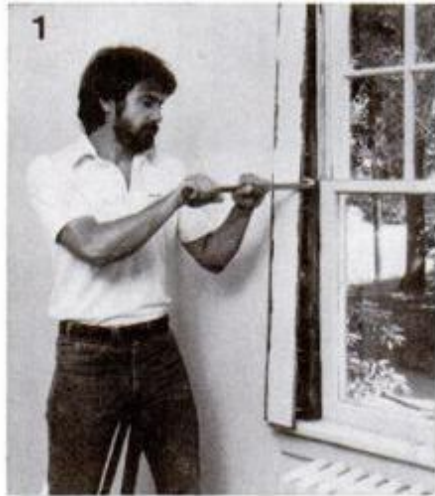
1 Flat pry bar neatly removes inside casing. If reusing trim, pull old nails through back of pieces with pliers.
