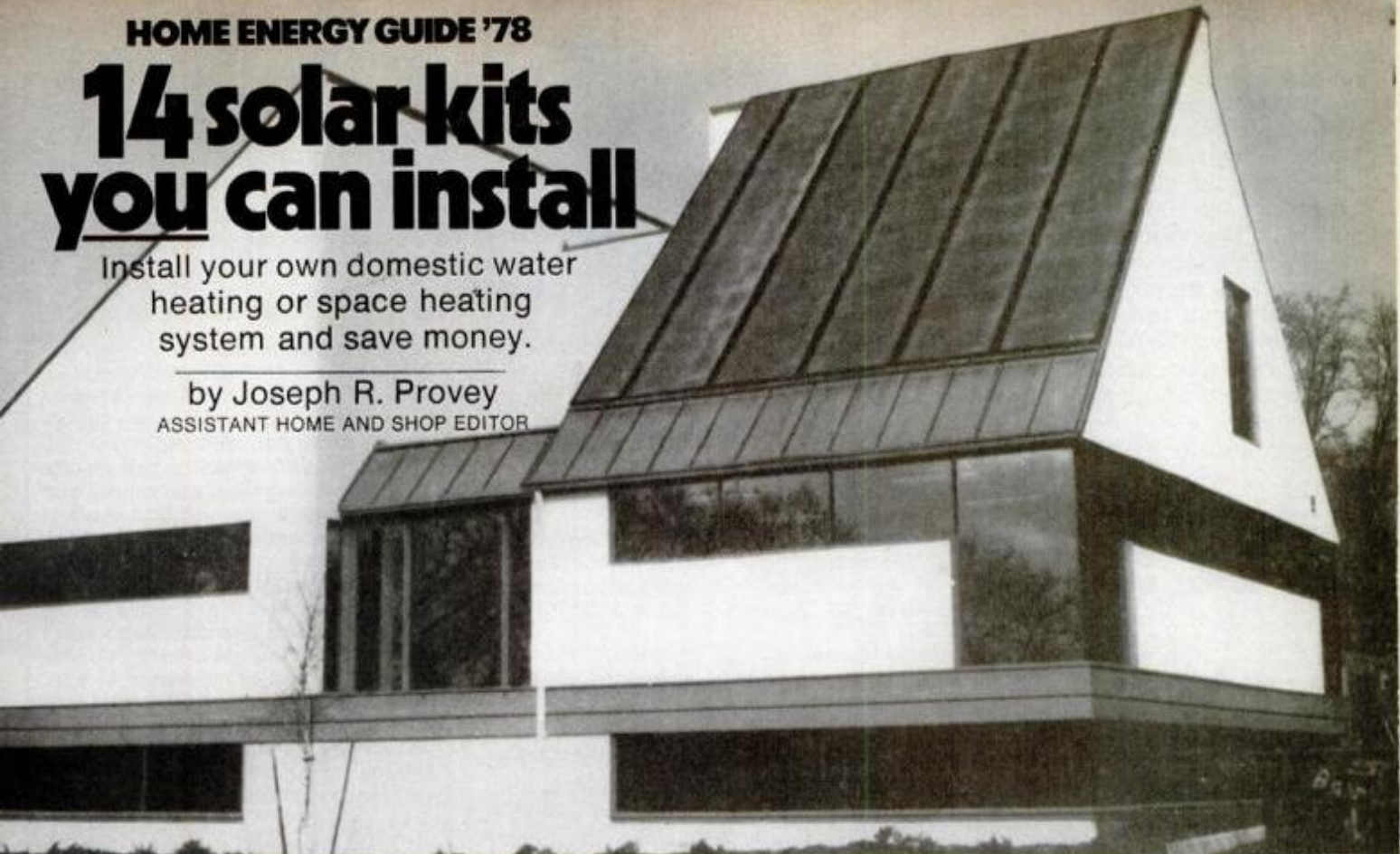
Nonmetallic collectors such as these by Calmac Manufacturing Corp. keep water-heating system costs under $1000.
