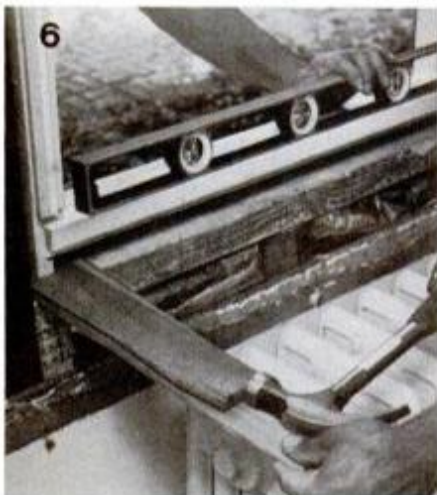
6 After inserting window, shim under jamb horns to level unit (see text). Helper steadies window, holds level.
