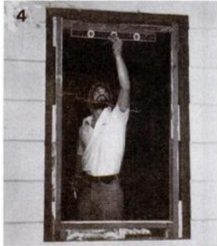
4 When needed, frame-in to recommended rough opening with spacer blocks, 2x4s. Stuff all voids with insulation.
