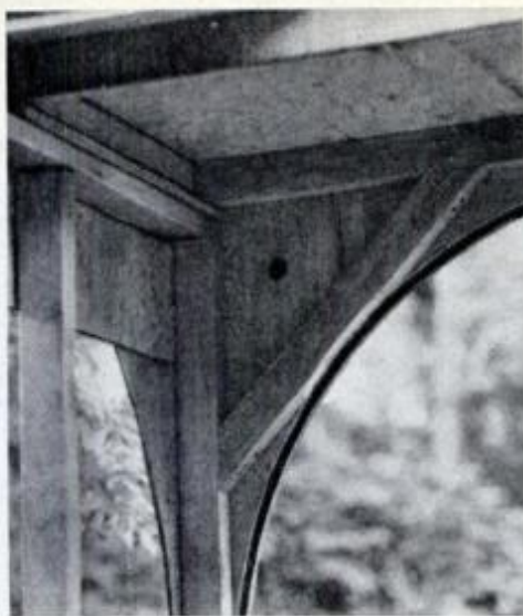
Diagonal braces add rigidity to the window walls. Cut 2x3s so that they fit inside the corners and are tangent to the circular cutout in the plywood.
