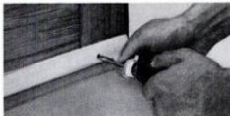
Screw-on-door-bottom strip stops drafts. Kit costs $2.94 from The Stanley Works, 195 Lake St., New Britain, Conn. 06050.
