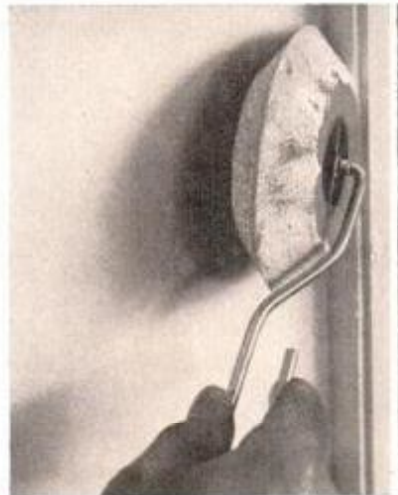
Foam roller is shaped for painting inside corners. Use to start job; then do trim with 3-in. roller, wall with 9-incher.
