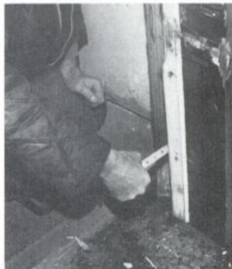
9 Measure distance from plumbed surface in several places for alignment.
