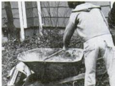
3. Pad uses 2½ bags of Sakrete mortar mix; after pouring add bricks (aggregate).
