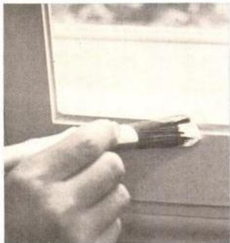
Oval sash brush is great for painting window trim—also mullions, scrollwork, moldings, any irregular surface.
