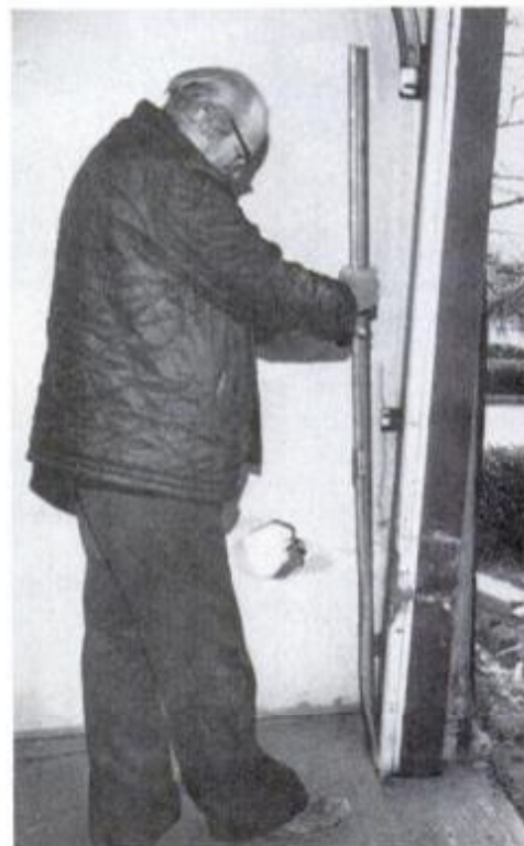
3 Next, twisted section of garage door track is unbolted; save hardware.
