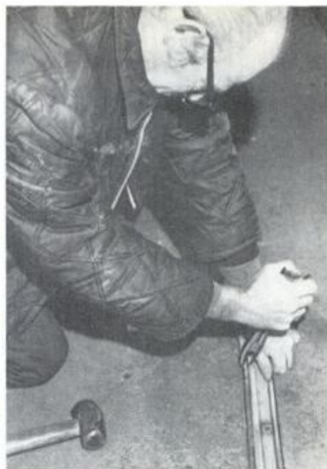
6 Heavy-duty pliers, muscle straighten the creased edges of the steel track.
