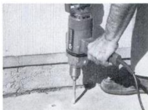
Bore masonry with a heavy-duty drill, carbide bit; use water to keep bit cool.
