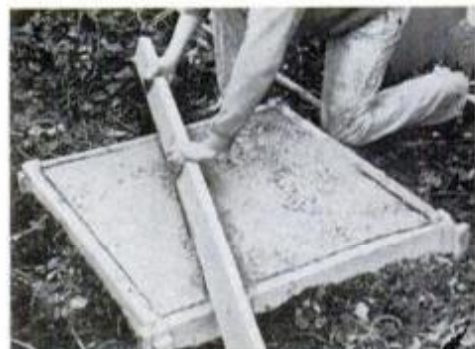
4. Level poured concrete by pulling 2x4 across forms with back-and-forth motion.
