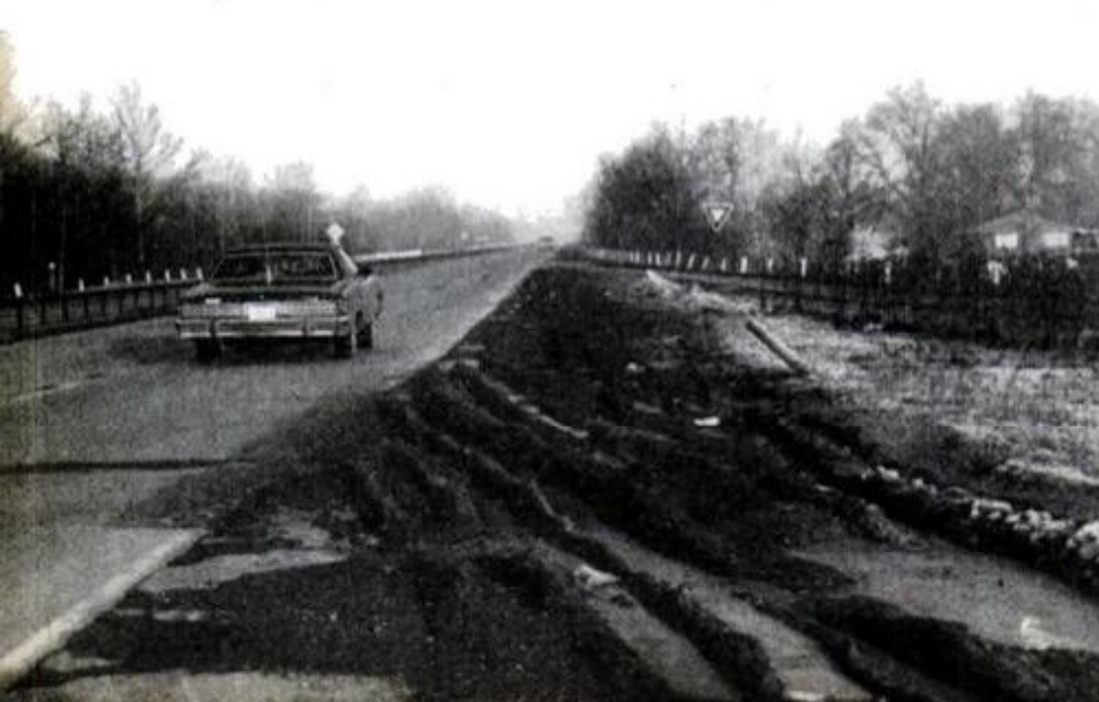
I-70 in West Virginia is a shambles of crater-filled shoulders. Lesser roads (right) like this in Connecticut, are in sad shape too.
