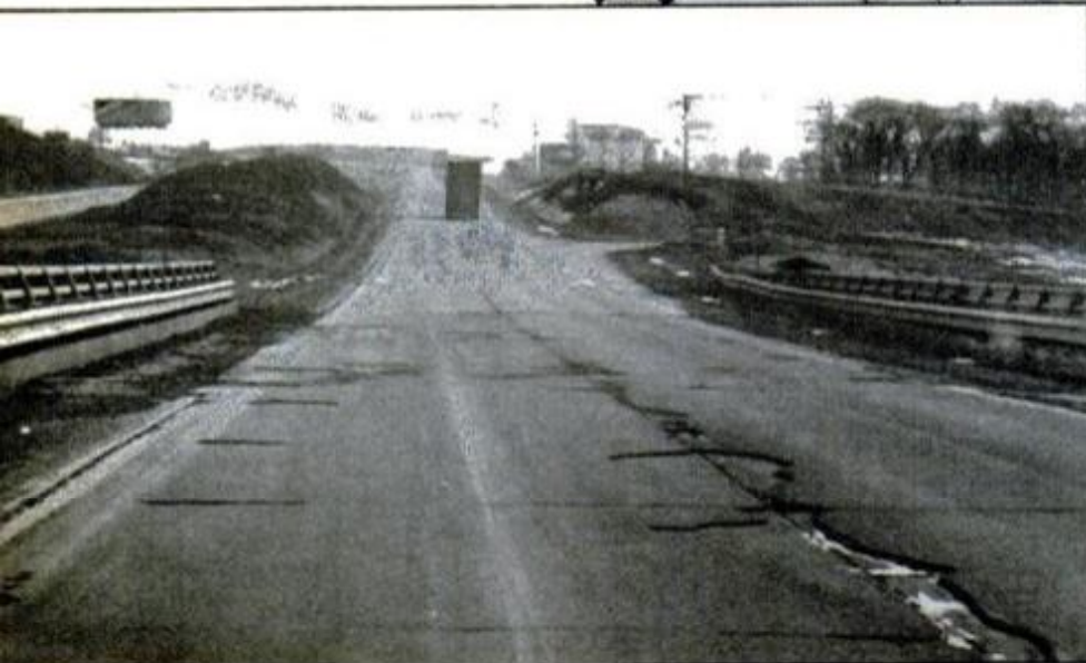
Thousands of highway bridges, pounded by excessive weights and speeds of today's trucks, are crumbling—like this one on I-81 not far from Shenandoah, Pa.
