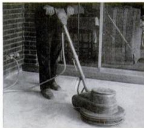
In cases of blistering and poor adhesion, answer is sanding, total refinishing.
