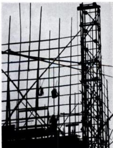
Towering bamboo caging is stronger than pipe scaffolds during typhoon season.
