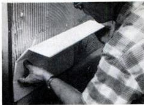
14 Mark pipe holes on tile. Test-fit by holding tile sheet in position.
