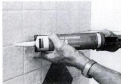
21 Grout all joints between sheets with same silicone used in sheets.
