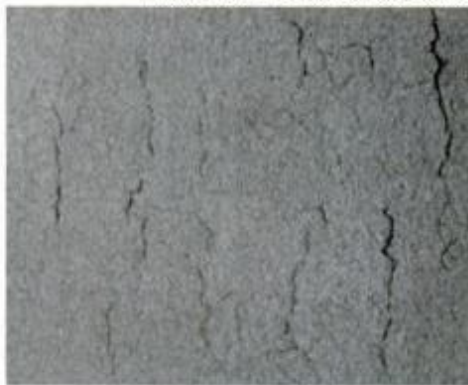
ALLIGATORING. Check-lines are usually due to hard paint on soft undercoat.
