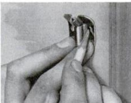
To hang fixture, start by marking pilot holes for the wall mounting plate.
