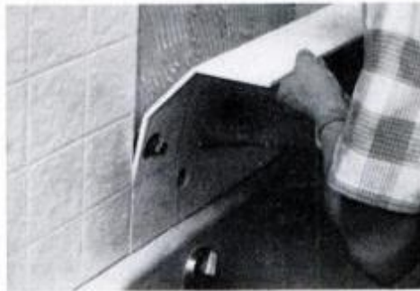
16 Install pre-drilled tile on wall and then replace the water pipes.
