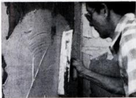
13 Remove pipes. Apply thin layer pre-sanded dry-set or latex cement.
