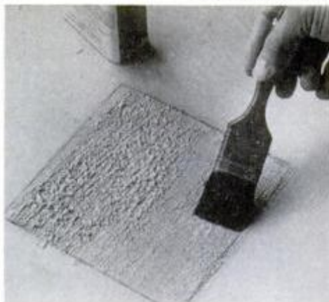
Cover area with any good commercial paint remover and let it sit until it acts.
