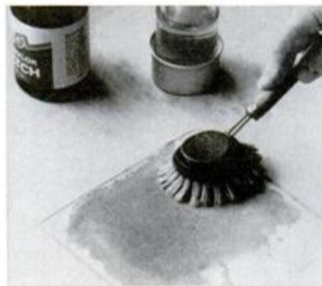
Cover exposed concrete with etching acid to extend scoring and rinse thoroughly.
