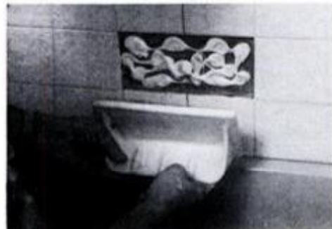
20 Apply silicone rubber liberally to Wonder-Board and install dish.
