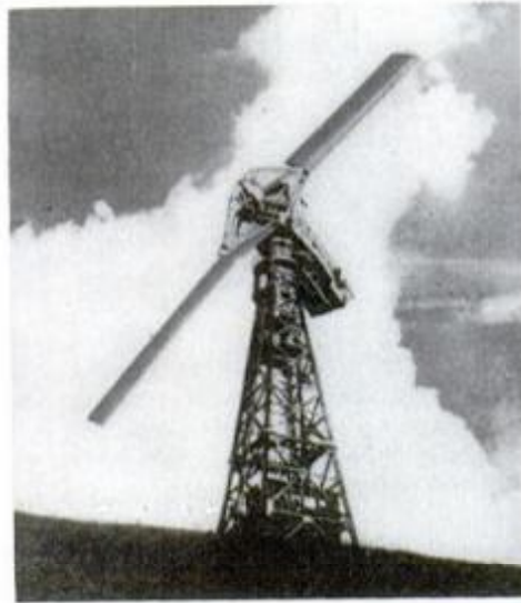
Built in 1940s, Smith-Putnam giant near Rutland, Vt., still holds record as largest windmill in world. It had 175-foot rotor, was damaged in storm and abandoned.
