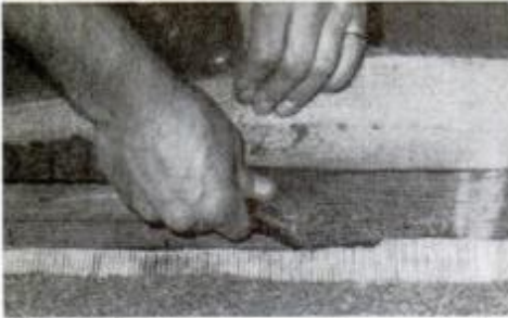
1. Trim old seam tape with razor knife. Remove pins in seams with screwdriver.
