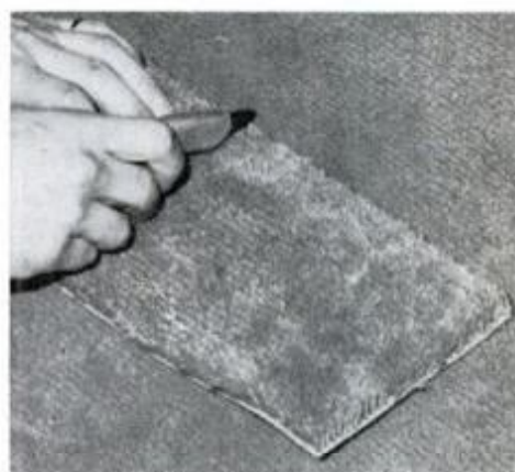
3. Align patch on bead already made as described in text; cut at 90° angle.
