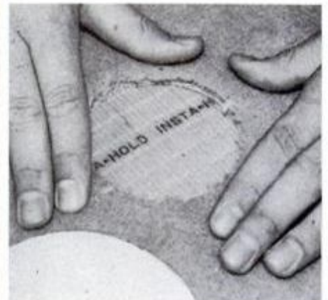
Position an adhesive disc underneath the carpet where the patch will be.
