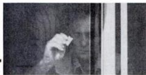
1. Scrape paint and dirt off the inside of window with a blade.
