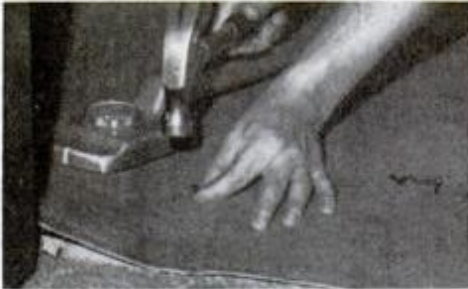
3. Tack both sides of carpet seam 3 in. from edge at 3-in. intervals.
