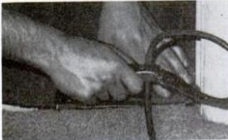
5. Staple or tack both sides of the tape. Secure seams with a special hot iron.
