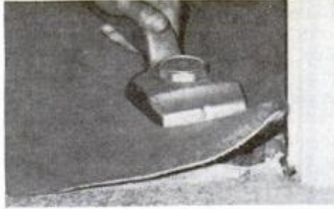
2. You can rent carpet kicking tool that removes excess stretch in the carpeting.
