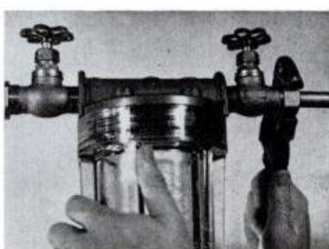
Now tighten locknuts. Both gate valves should be closed at this point.
