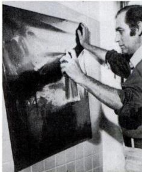
5. Wet adhesive side of film. Static electricity holds it to tile for spraying.
