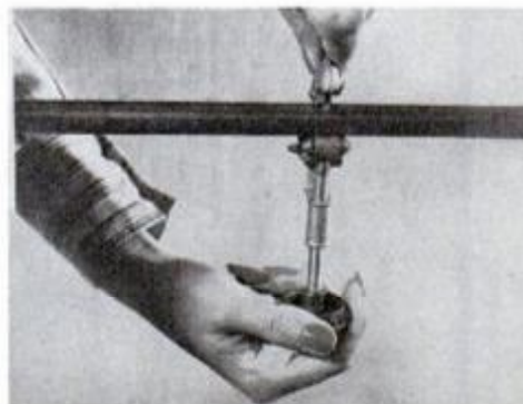
Shut off water, drain pipes, then remove length of pipe specified by filter maker.
