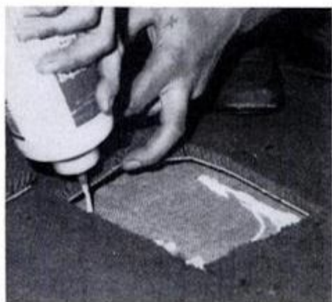
7. Squeeze carpet latex adhesive evenly on the support; avoid the surface carpet.
