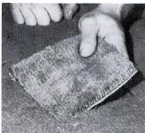
8. Make sure pile direction is correct and carefully place the patch into the hole.
