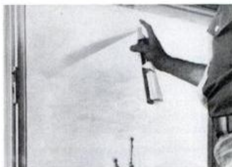
4. Wet down the window with a water spray bottle: use plenty of water.
