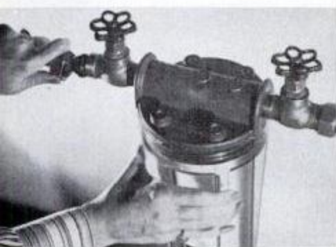
Place the filter in position, with the inlet on the water-meter side of the line.
