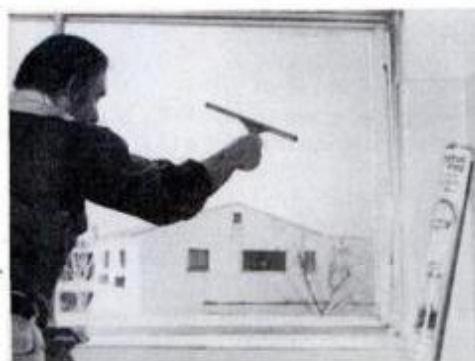
2. Thoroughly clean window with clear water. Squeegee away excess moisture.
