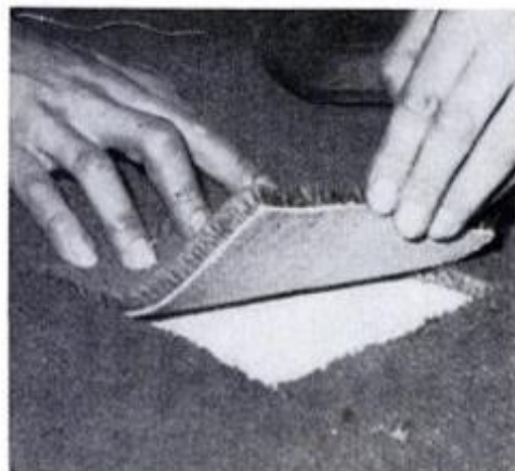
4. Cut along bead, grasp the old carpet and finish cutting to remove burn area.
