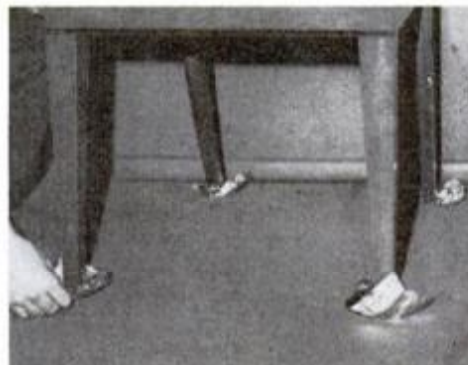
Place aluminum foil under furniture so wood stain won't bleed to moist carpet.
